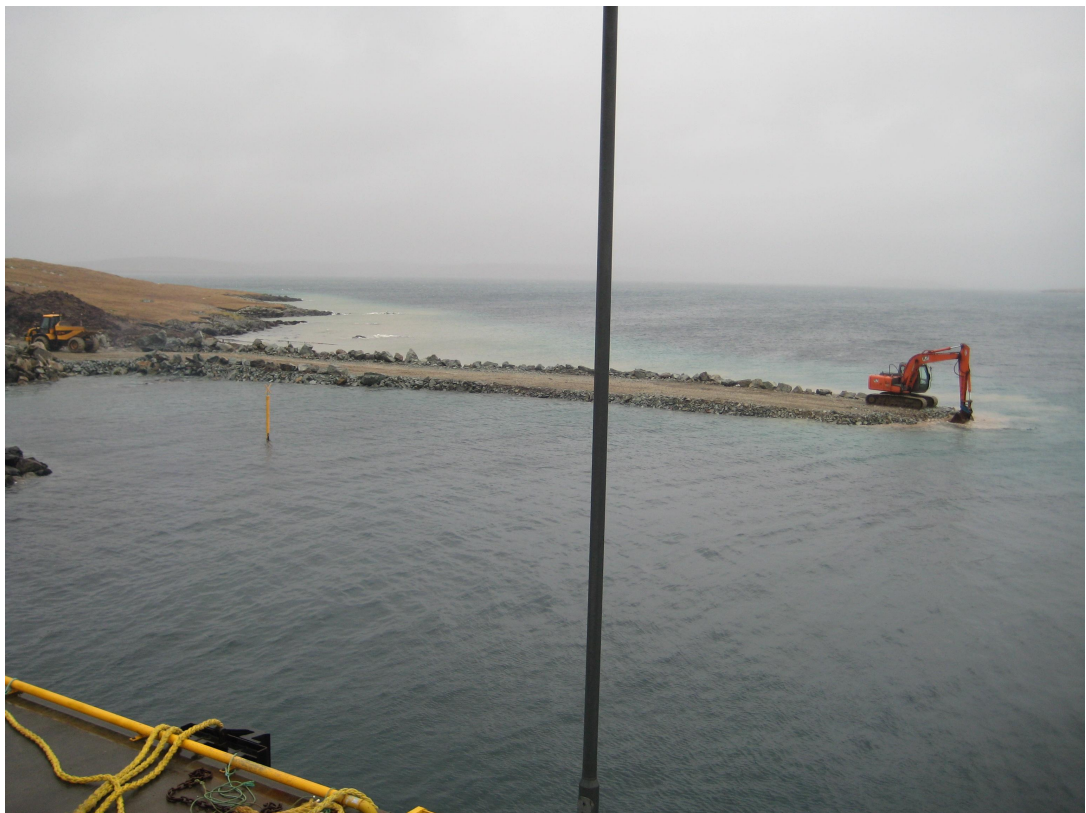
Recent picture of progress on building breakwater
