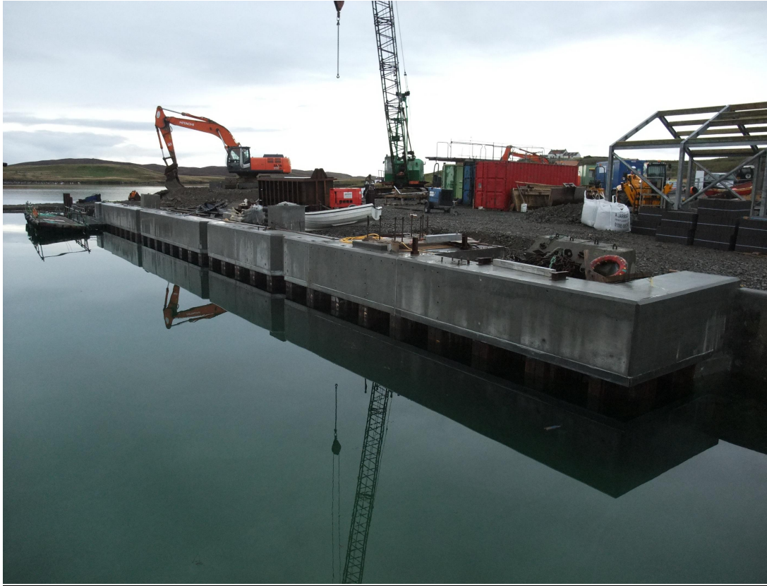
1. View on inner quay face showing completed concrete capping beam.
