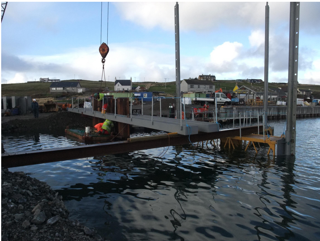
2. Work continues on outer leg of pier, with pile guides in position and first piles driven.
