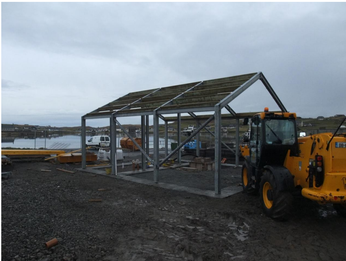
3. Foundations and frame for Ferry Terminal waiting room.
