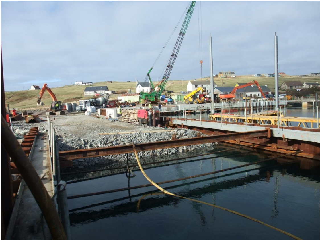
3. View from end of seaward leg of the pier, with piles in position and infill progressing.
