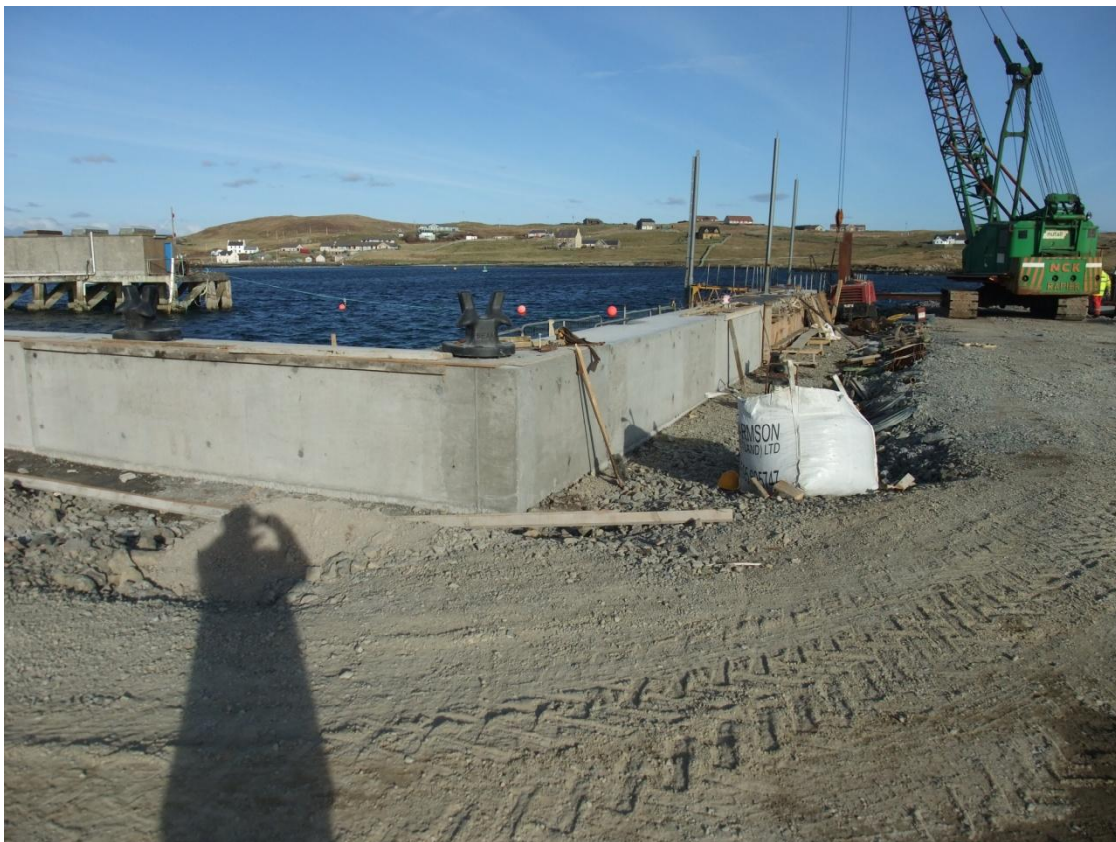
4. View over seaward leg of pier with capping beam and bollards in place.
