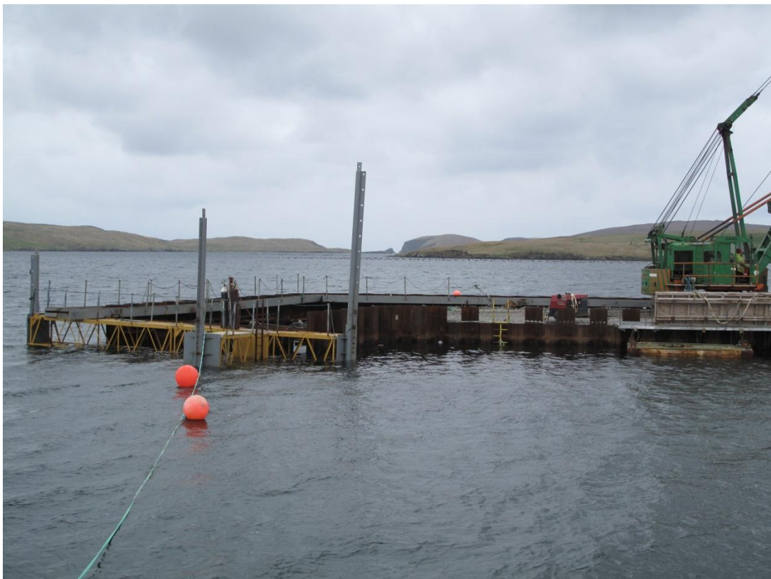
2. Work continues on piling the outer end of the finger pier.
