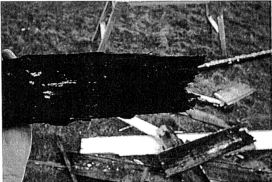
Photo showing the extent of the rot in the annex planking the planking in place was so rotten that it absorb water like a sponge During freezing temperatures the water would soak the fibre insulation and freeze against the inside walls making it almost impossible to heat the annex rooms sufficiently for comfort
