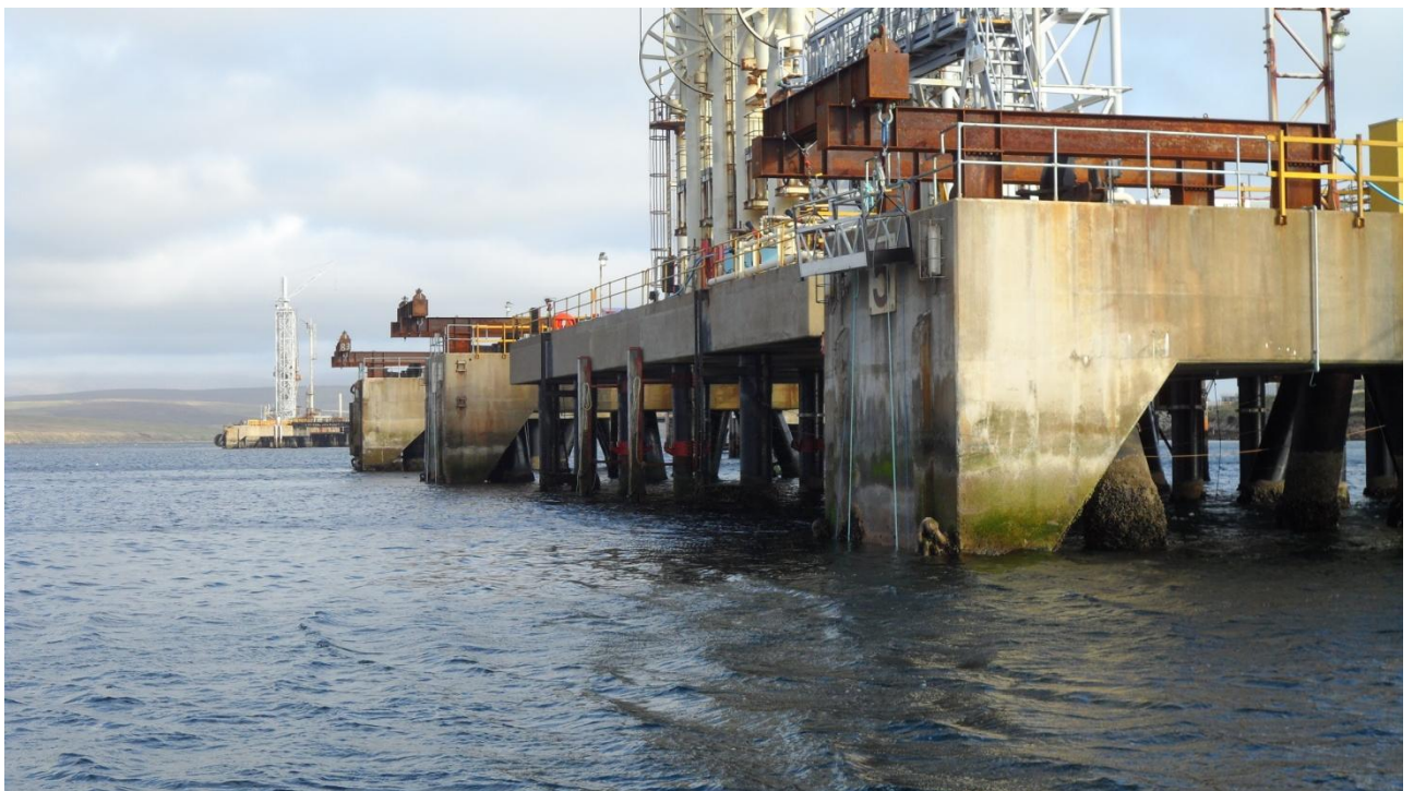
4. Dolphins with original fenders removed, ready for new fender preparatory works
