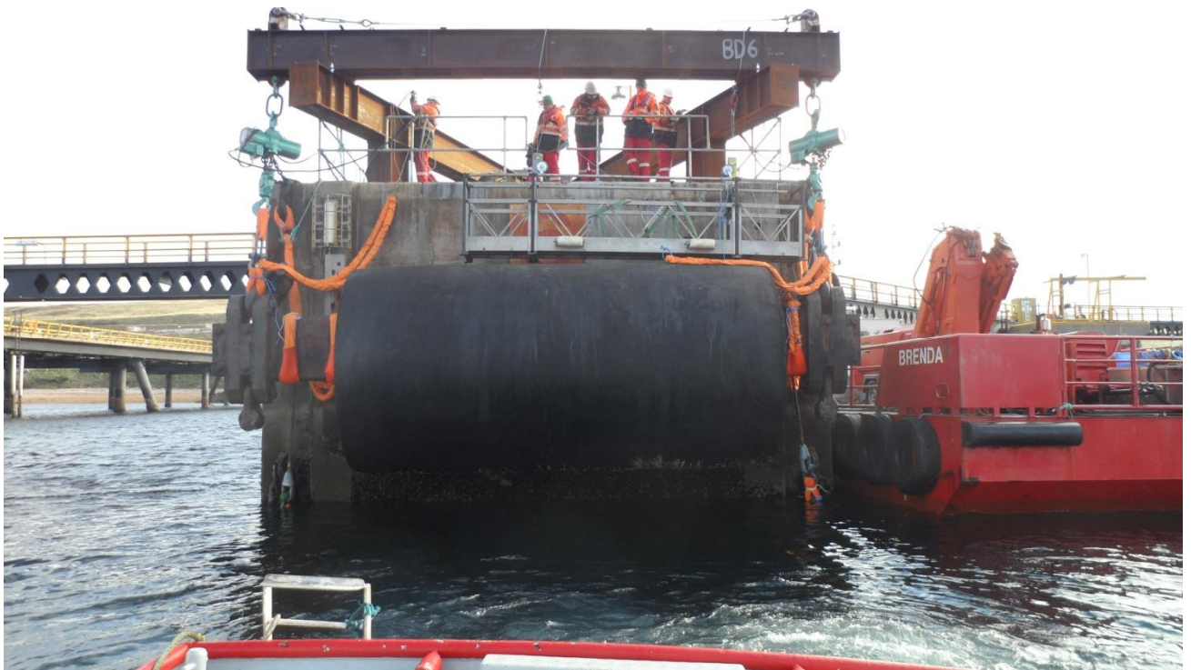
3. Old fender being lowered from face of dolphin.
