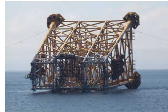
First of Clair Ridge jackets awaiting installation by Heerema's Thialf .
