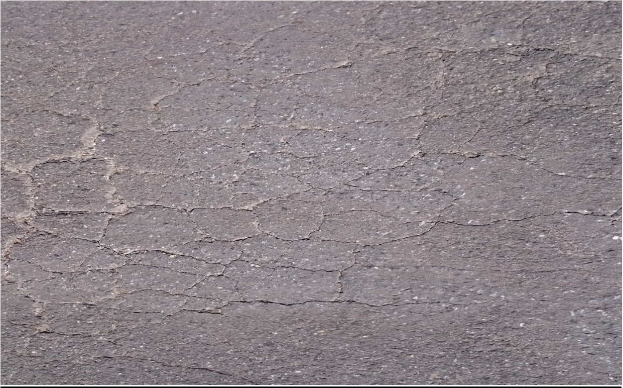
Cracking at North End of Runway
