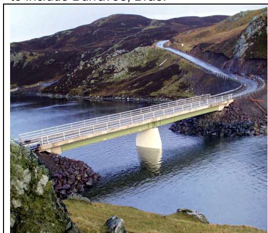
Muckle Roe Bridge.
