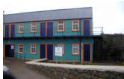
North Ness – Restored Gutter's Hut
