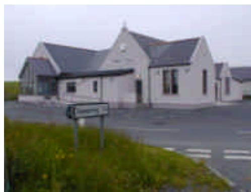
The newly refurbished Lunnasting Hall, Vidlin
