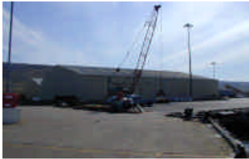
Blackness Pier's New Cargo Shed
