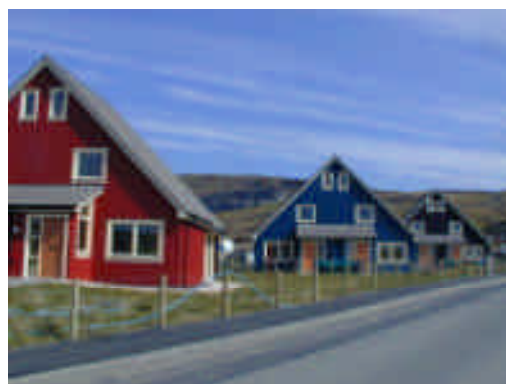
New HHA Housing at East Voe
