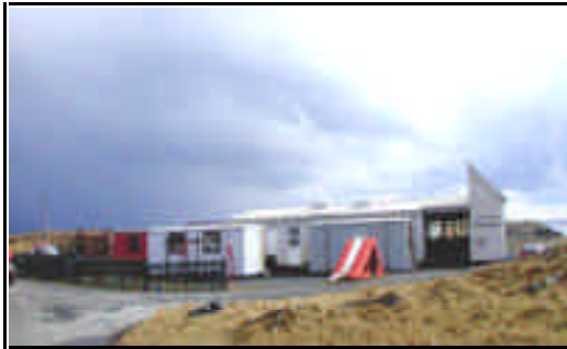
The existing Skerries School
