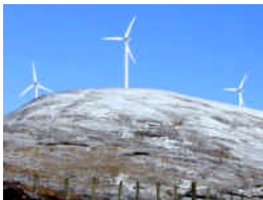
Aerogenerators at Burra Dale
