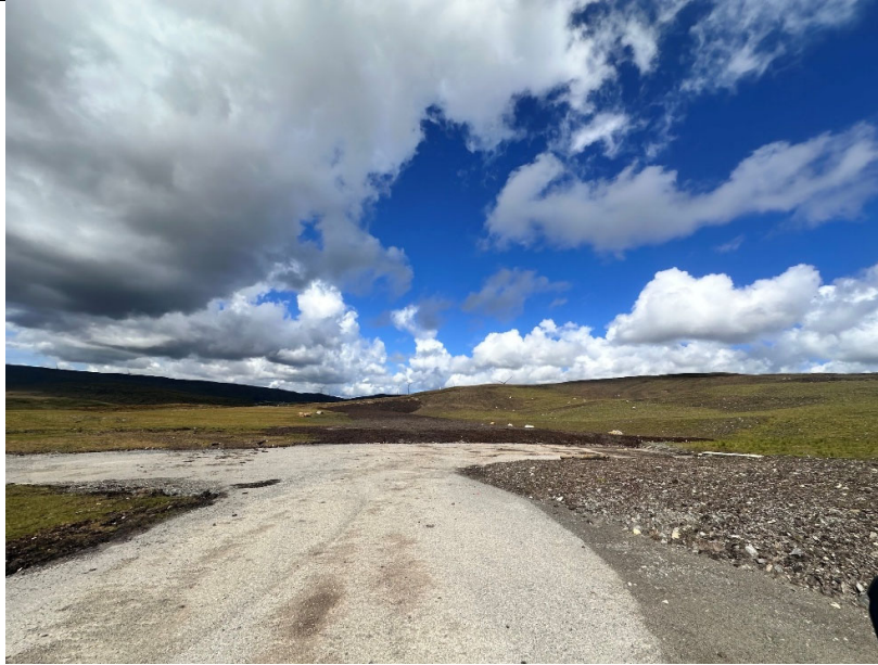
Photo 9. Main Compound reinstatement
