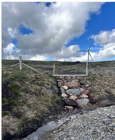
Photo 12. Drainage at T076 downstream from NBP05
