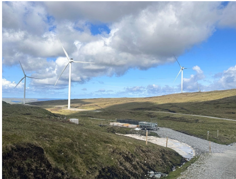
Photo 7. Vegetated slopes and backfilled cut off ditches north of KBP02
