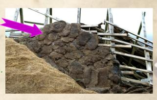
4. Now gather your gloy (thatching straw) together into bundles. Place the bundles of straw on the turf, making sure you keep an equal thickness over the entire roof.
