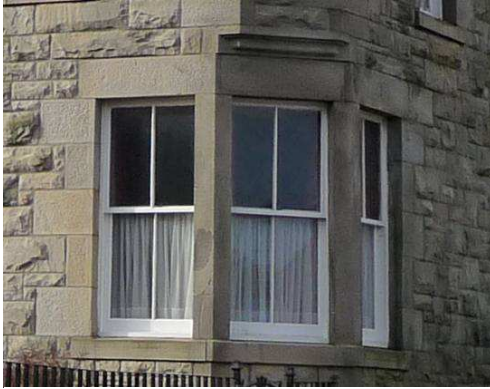
Windows are traditionally timber sash and case, painted white.
