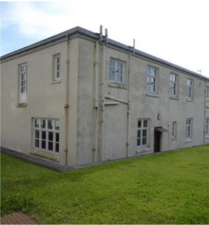
The external walls of the building are covered with masonry paint, which imposes a rather costly ongoing maintenance burden. This paint is beginning to show signs of deterioration and redecoration will be required in the relatively near future. It should be noted that many masonry paints inhibit breathability of the building fabric and consideration should be given to using a vapour permeable mineral-based or similar coating in the future.
