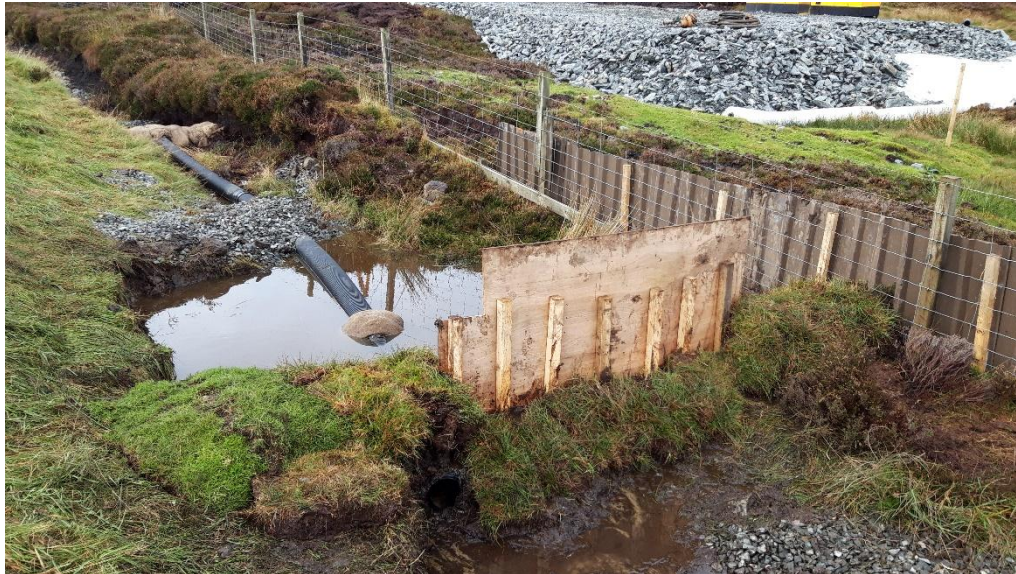
Photo 3. View of ponded groundwater due to be pumped back to settlement pond.
