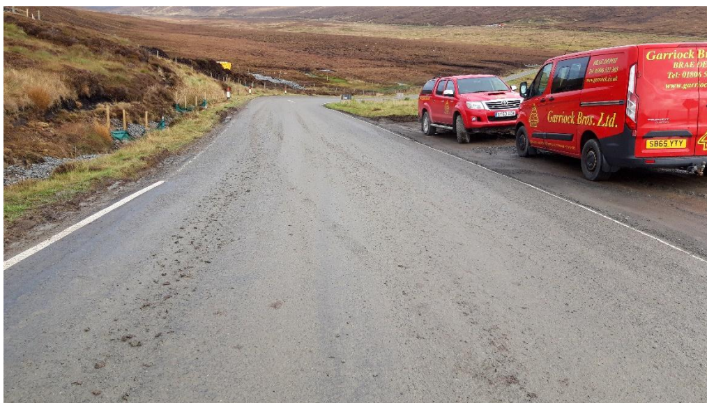
Photo 6. Mud observed on road at the temporary access point to Sandwater Road compound
