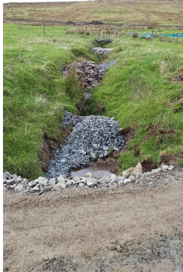
Photo 9. View of Burn of Weisdale tributary containing silt fencing and stone check dams following incident on 1 st October 2020.
