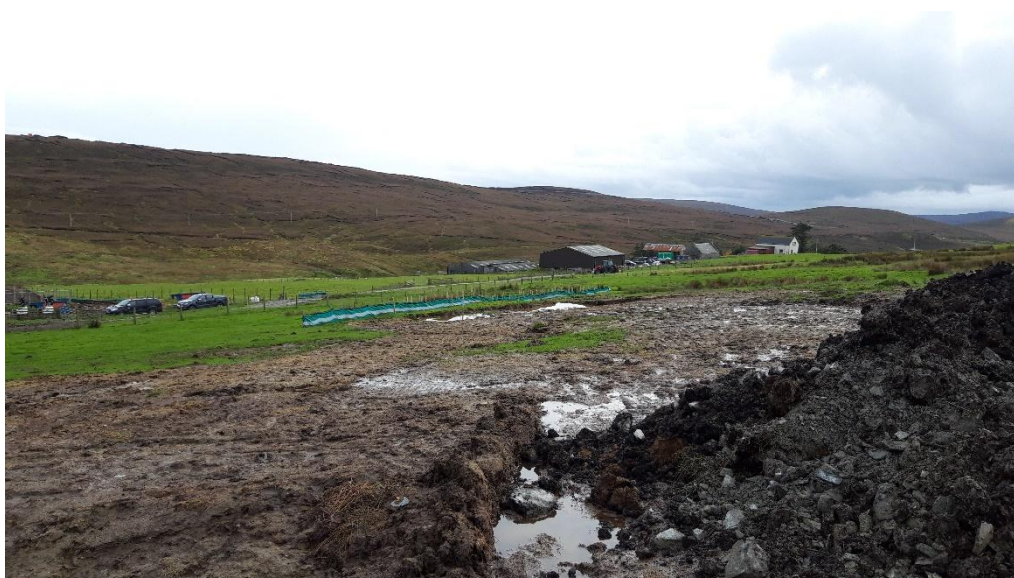
Photo 8. View of silt fencing beyond settlement pond, downgradient of the Kergord Access Track.
