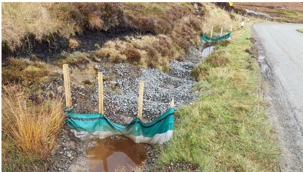
Photo 5. Example of silt fences and clean stone in place to aid drainage in ditch to south of construction area on Sandwater Road
