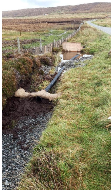
Photo 4. View of pipe placed in drainage channel to allow surface run-off to by-pass ponded groundwater.
