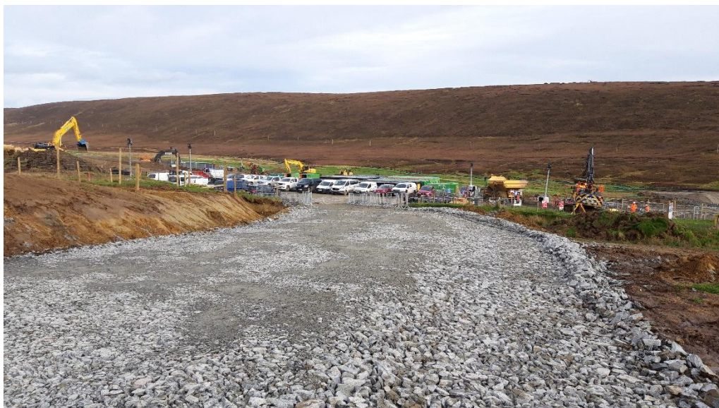
Photo 10. End of Kergord Access track with filter drain on right hand-side of image, reportedly constructed to manage run-off that would otherwise flow towards BAM Construction compound in the distance.
