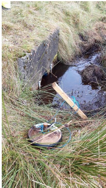
Photo 1. Plug attached to wooden stake at Culvert 3
