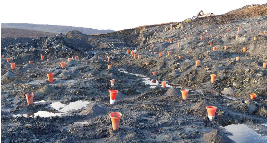
Photo 16. Ground prepared for blasting in Main Compound
