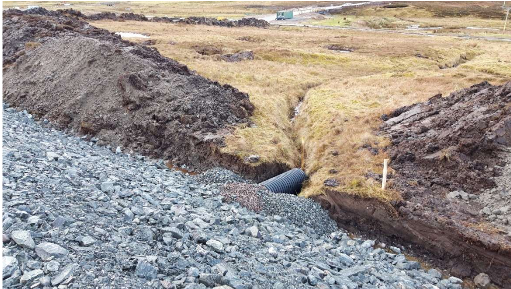
Photo 7. Example of culverted watercourse beneath new Sandwater road
