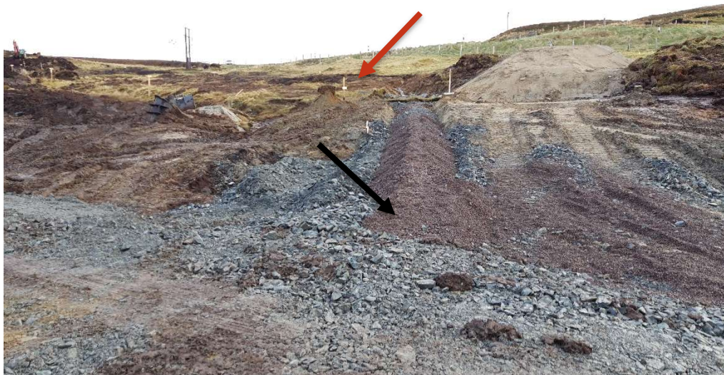
Photo 5. Burn of Swirtars culvert (marked by black arrow) and channel realignment (marked by red arrow) on the upgradient side of Sandwater Road construction.
