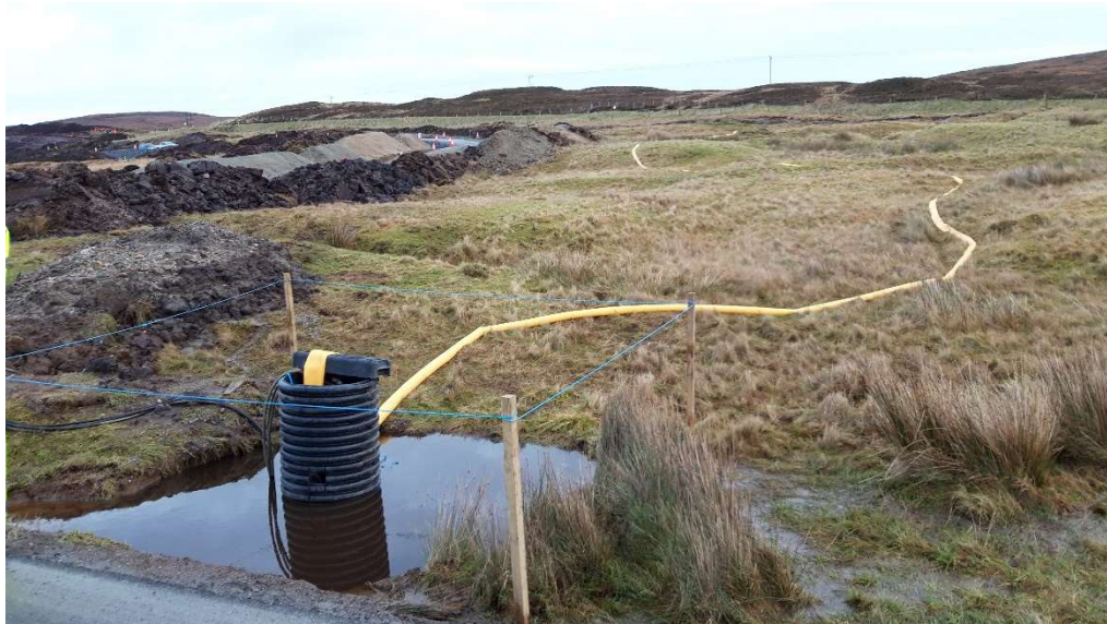
Photo 9. Sump at western end of Sandwater Road with pump and pipe to divert water back to settlement pond
