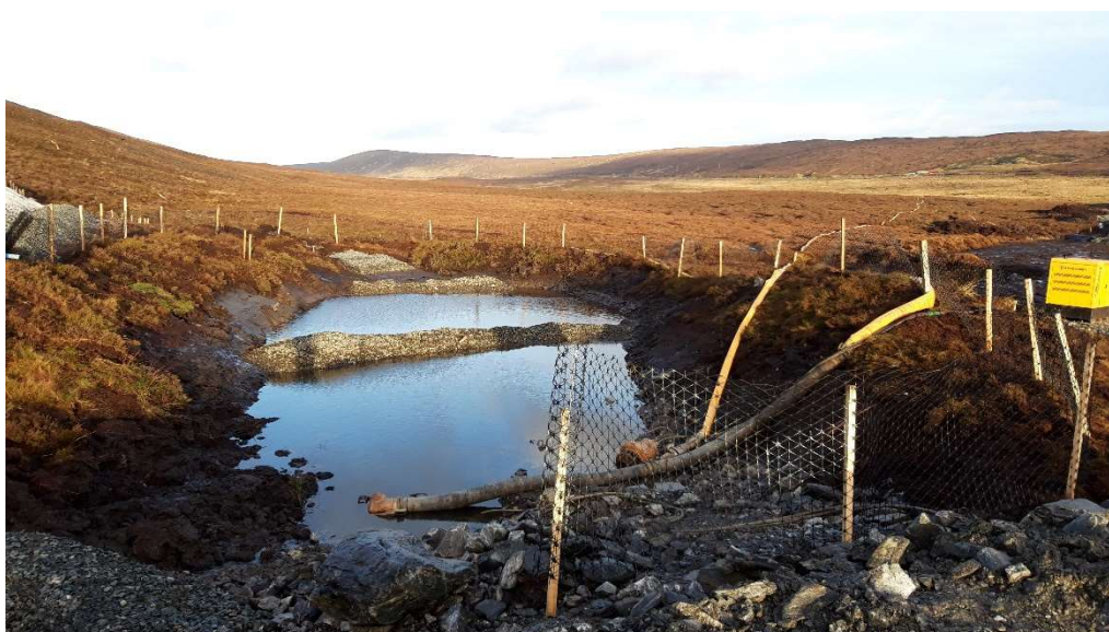
Photo 12. Settlement pond at Sandwater Road. Pump and yellow pipes used to re-divert clean water back to the wider catchment area.
