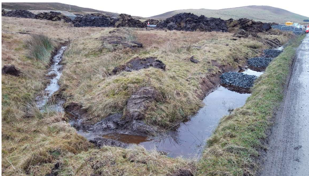
Photo 8. View of drainage channel with check dams diverted towards sump in the distance.
