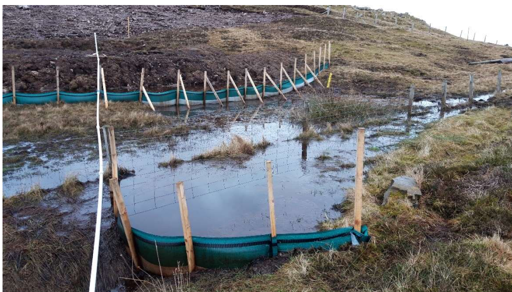
Photo 2. Silt fencing in drainage channel upgradient of culvert at Scord of Sound
