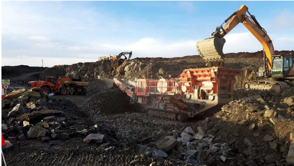
Photo 13. Use of mobile plant for crushing at Sandwater Road.
