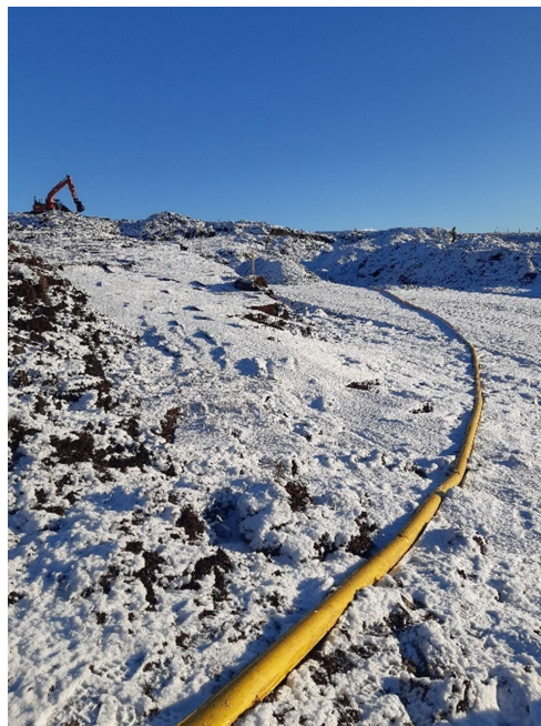
Photo 4. Hose used to divert silty water from the Upper Burn of Swirtars to settlement pond
