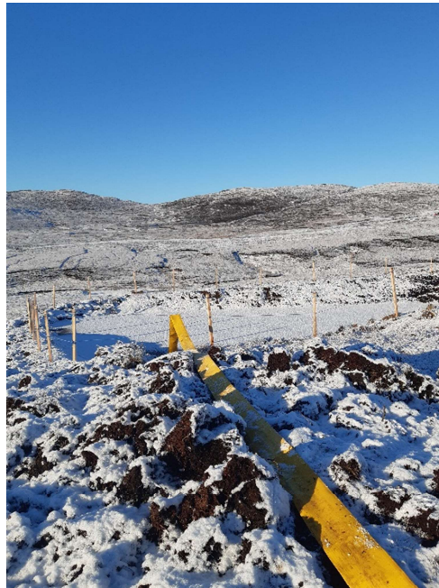
Photo 5. Hose used to divert silty water from the Upper Burn of Swirtars. Settlement pond delineated by posts and frozen at the time of the audit.
