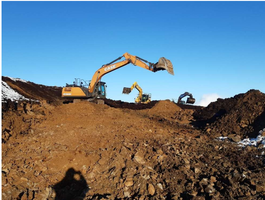
Photo 1. Excavators at Spur 5, peat and mineral soils cast to the side of the track
