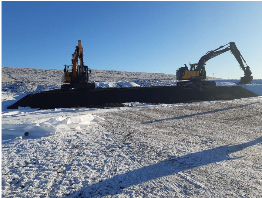
Photo 9. Eastern end of Sandwater Road, excavators placing LECA clay aggregate on new road surface
