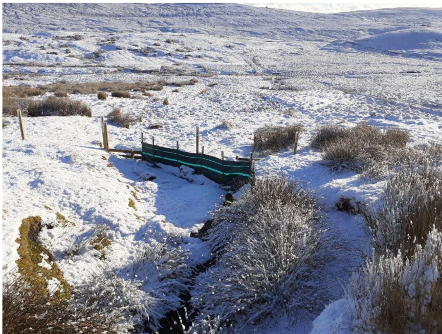
Photo 2. New silt fencing east of KAT Ch.1300 to divert dirty water from peat pipe. (Photograph originally appended to RJM Environmental Incident Report Form ENV 005, dated 26 th January 2021).
