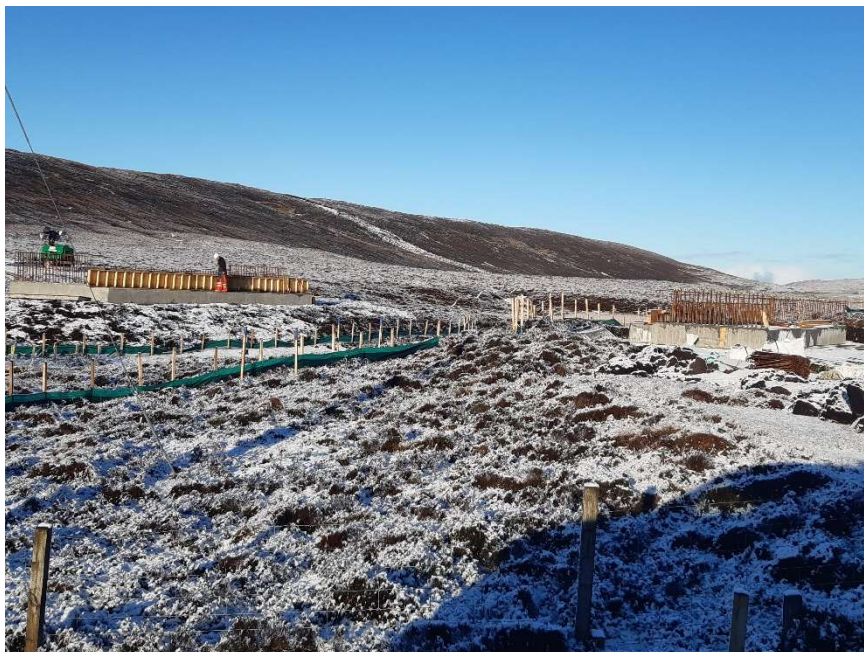
Photo 10. Bridge abutments on the banks of the Burn of Pettawater. Silt fencing has been erected on both banks.
