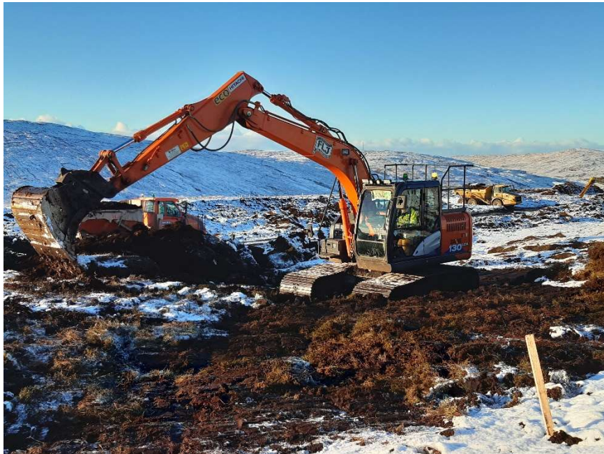
Photo 14. Excavators and dump trucks operating in peat restoration area P0809.
