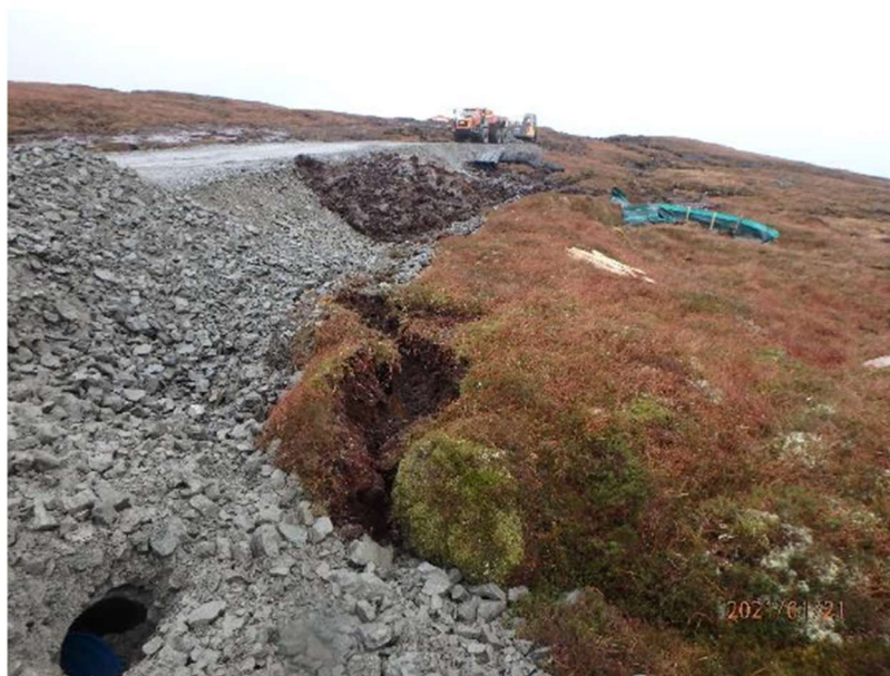
Photo 18. Area of damaged culvert (reported in NCR on 22 nd January 2021) following bearing failure on Spur 22.
