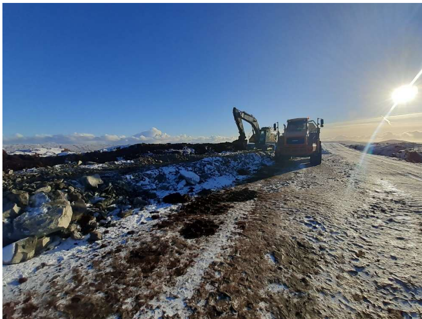
Photo 12. Excavator forming the hardstanding for crane pad at K86 on Mid Kame Ridge
