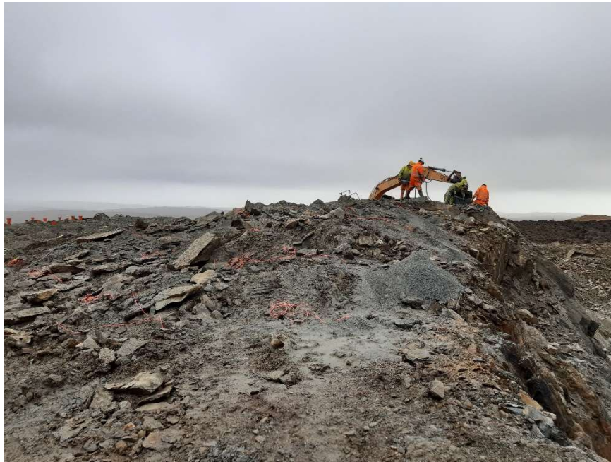
Photo 3. Progress at Borrow Pit KBP02. Foreground of image shows drilled areas prior to blasting.
