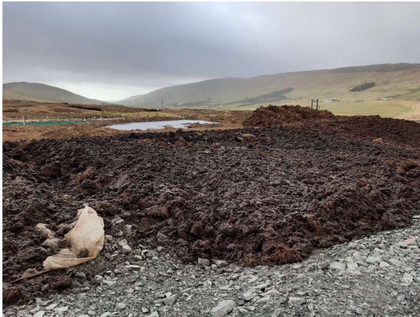
Photo 6. Ongoing soil reinstatement at CH.1400 of Sandwater Road.
