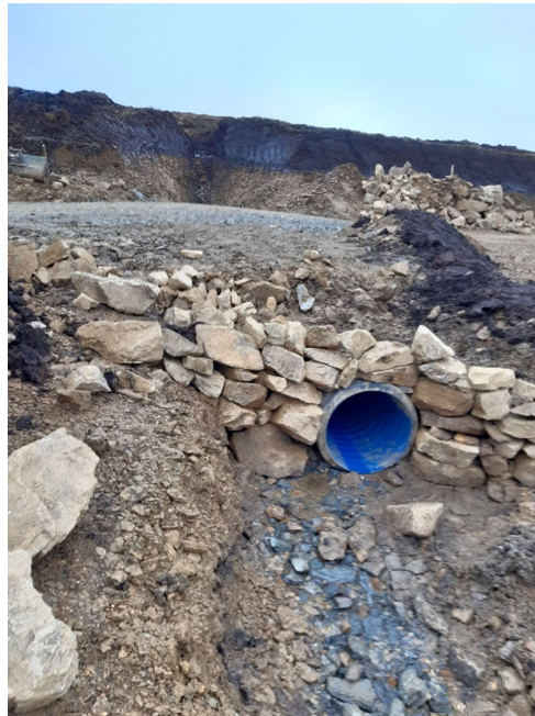
Photo 1. Clean water culvert installed under the track at Spur 5 (Kergord).
