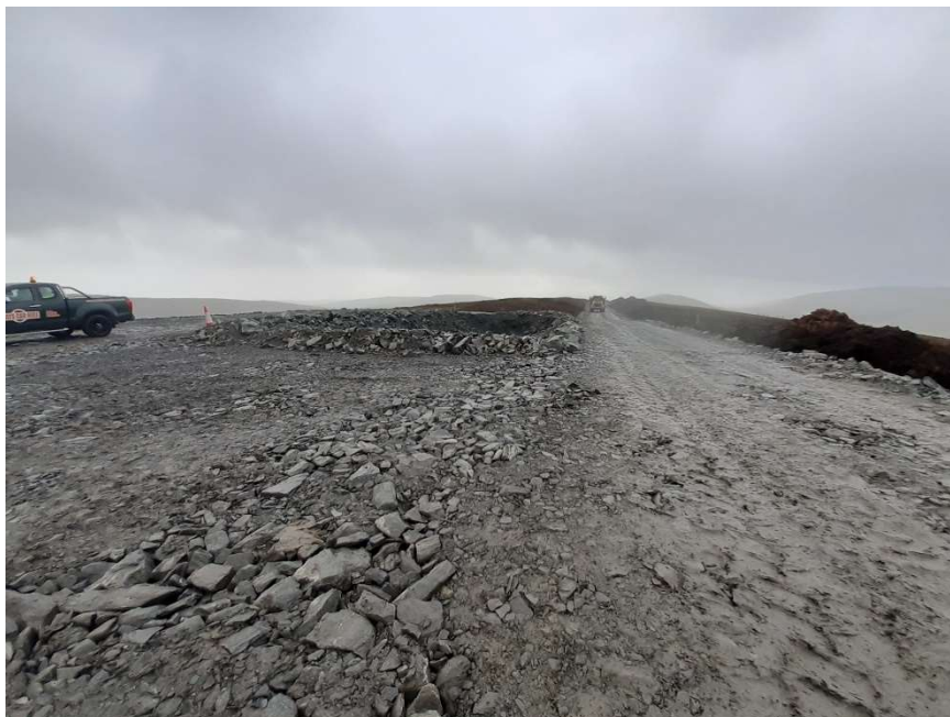
Photo 10. Crane hardstanding that has been formed at K86.
