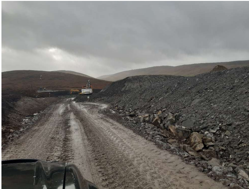
Photo 9. Mineral soil stockpile at the southern end of Mid Kame Ridge. Material is being used to form access tracks.
