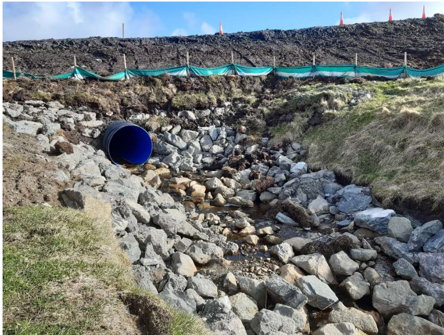
Photo 1. Droswell Burn culvert beneath Kergord Access Track
