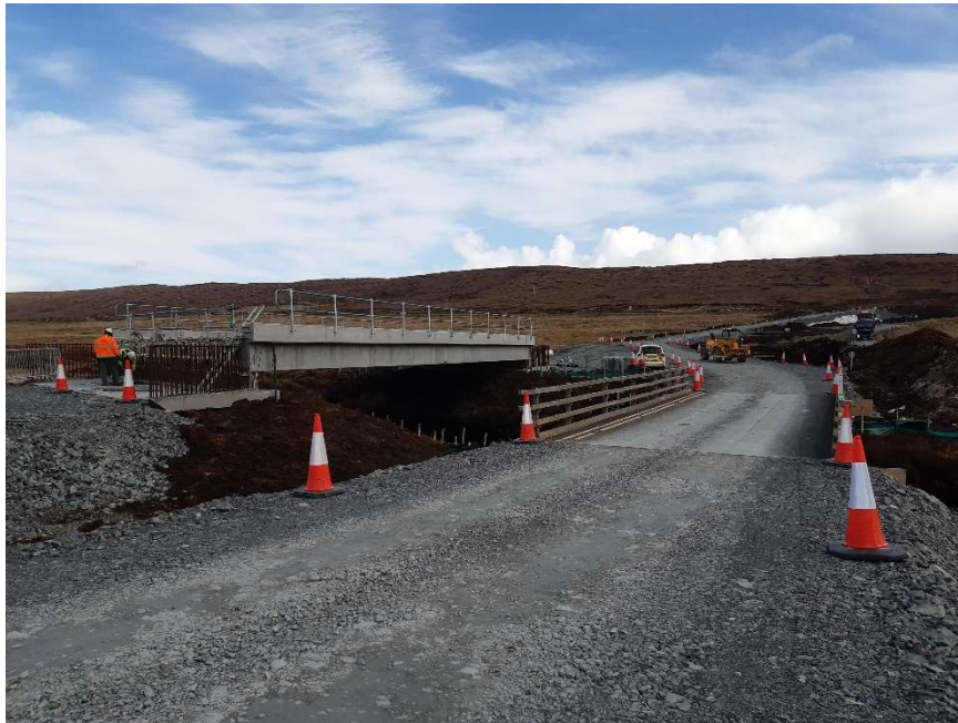
Photo 7. Temporary bridge over the Burn of Pettawater shown on the right. Permanent bridge, under construction, located immediately to the left.
