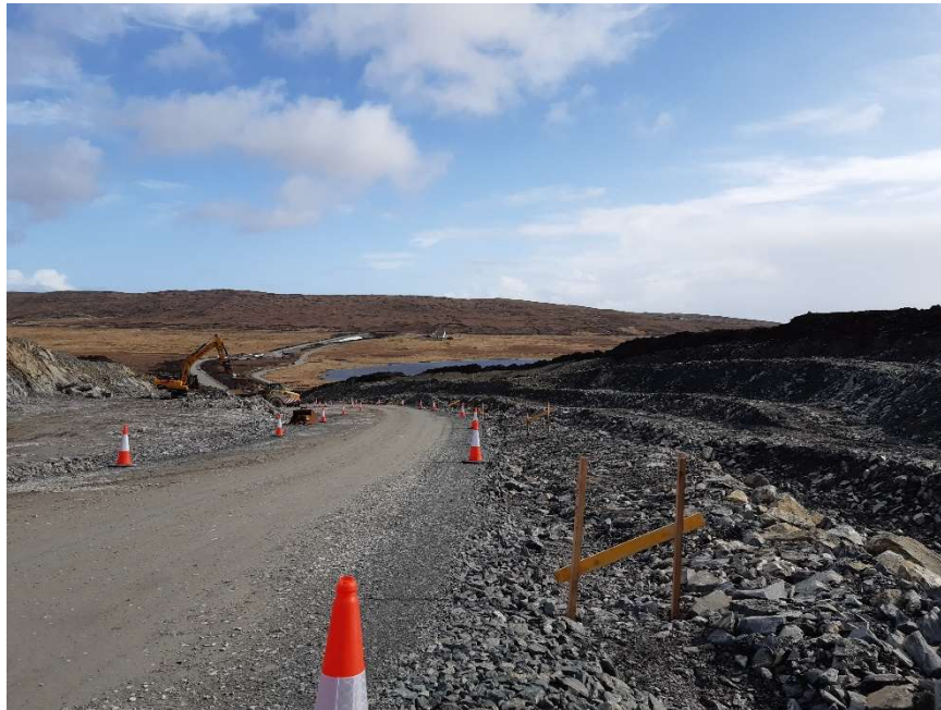
Photo 5. Reprofiling of verge on Sandwater Road.
