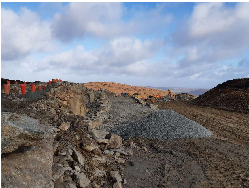
Photo 2. Access to borrow pit KBP02. Area prepared for blasting is shown on the left hand side of the image.
