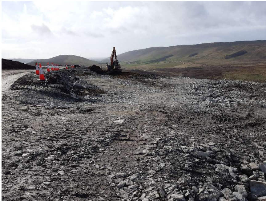
Photo 9. K88 Hardstanding crane pad.
