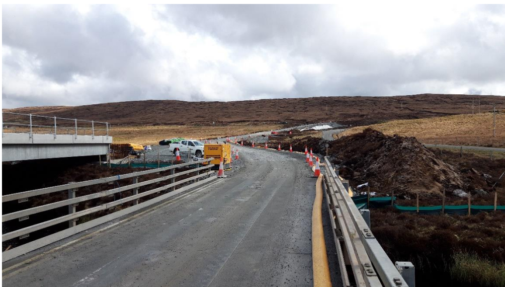
Photo 6. Dust mitigation measures ready for use as required along Sandwater Road
