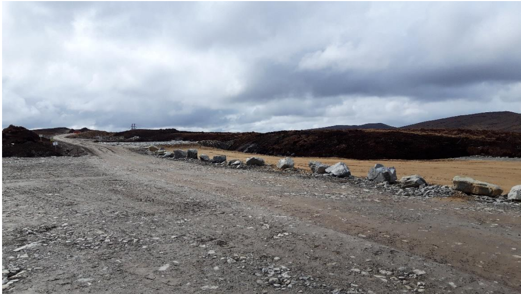
Photo 7. View of peat restoration area P08 from K79 crane pad hardstanding
