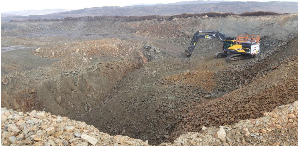
Photo 15. Excavator progressing extraction of rock within borrow pit NBP05.
