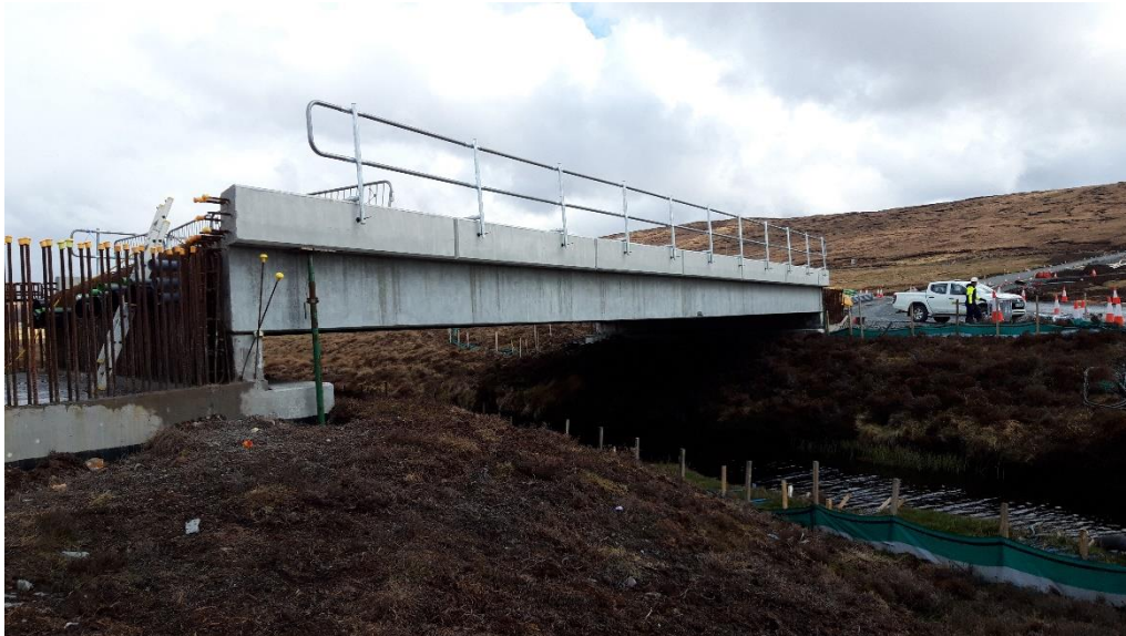
Photo 5. Progress with construction of permanent bridge over the Burn of Pettawater
