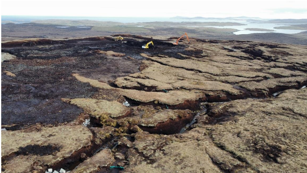
Photo 17. Aerial view of peat restoration area P27.
