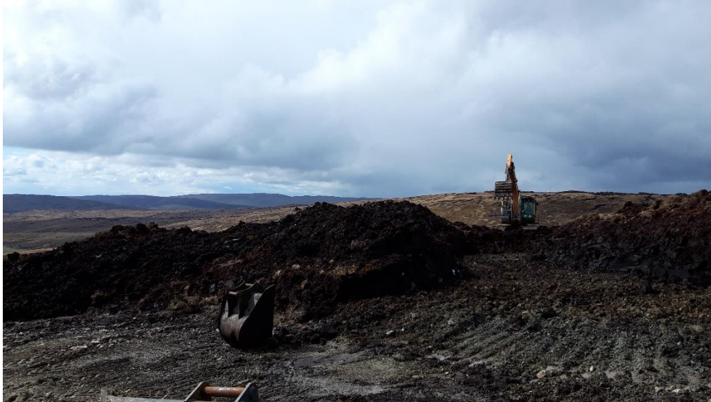
Photo 13. Excavation of peat at the location of N132 on Spur 32.
