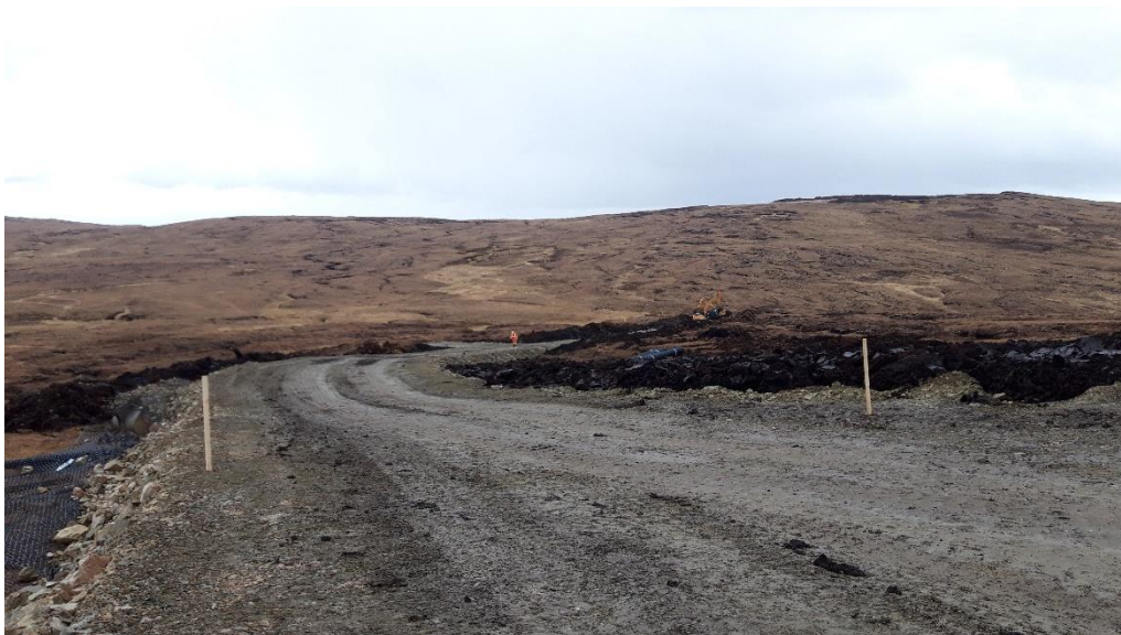
Photo 14. View of progress along Spur 27, viewed from Junction 28.
