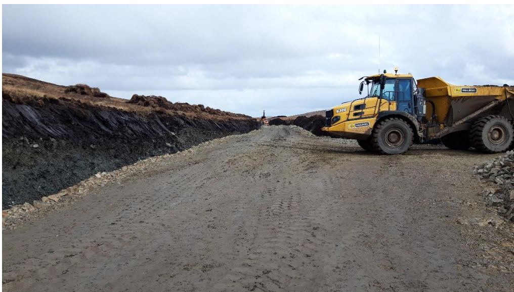
Photo 12. Progress of track construction at Spur 32 towards N137.
