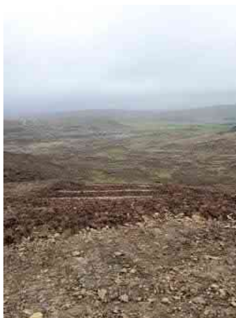
Photo 4. Remediated peat slip area at CH2450 of Spur 4 at Kergord.
