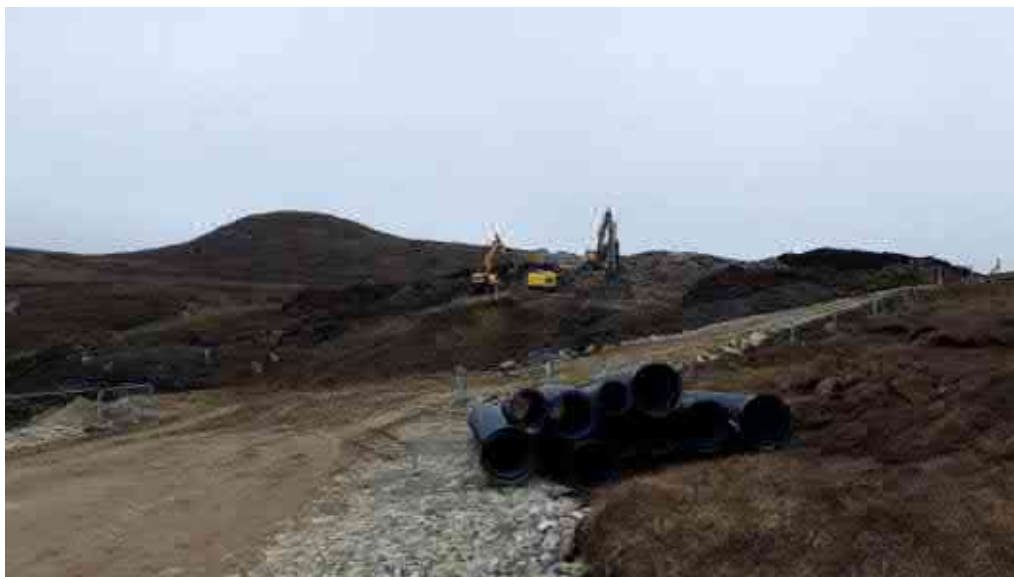
Photo 3. Area to be drilled and blasted to allow creation of final access track on Spur 4. Temporary pilot track has been constructed (on right hand side of image).
