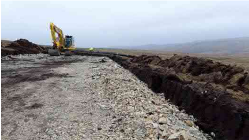
Photo 15. Construction of access track on Spur 27.
