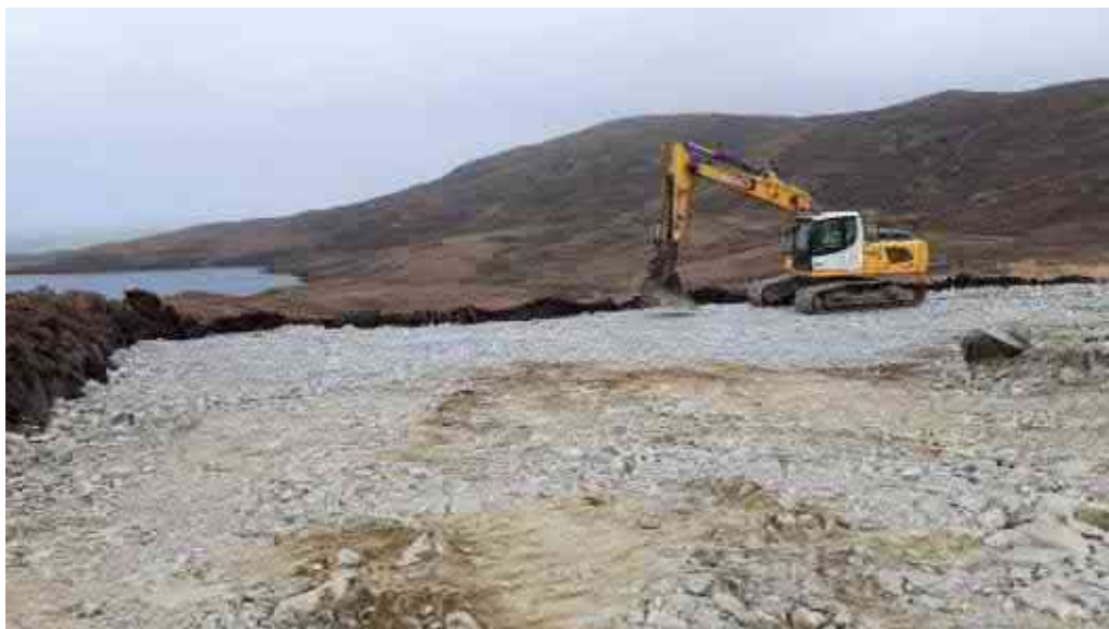
Photo 2. Formation of hardstanding crane pad at turbine K60.
