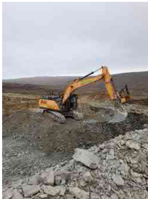
Photo 14. Extraction of rock to create access to turbine N129 and associated hardstanding.
