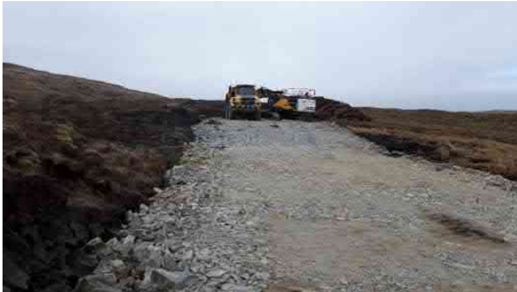
Photo 1. Removal of peat and placement of stone on access track on Spur 4.
