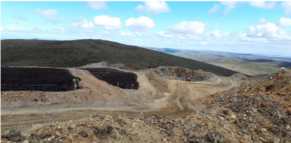
Photo 4. View of KBP02 and the adjacent peat restoration areas. Blasting had taken place at KBP02 since the previous audit exposing rock better suited to road capping.
