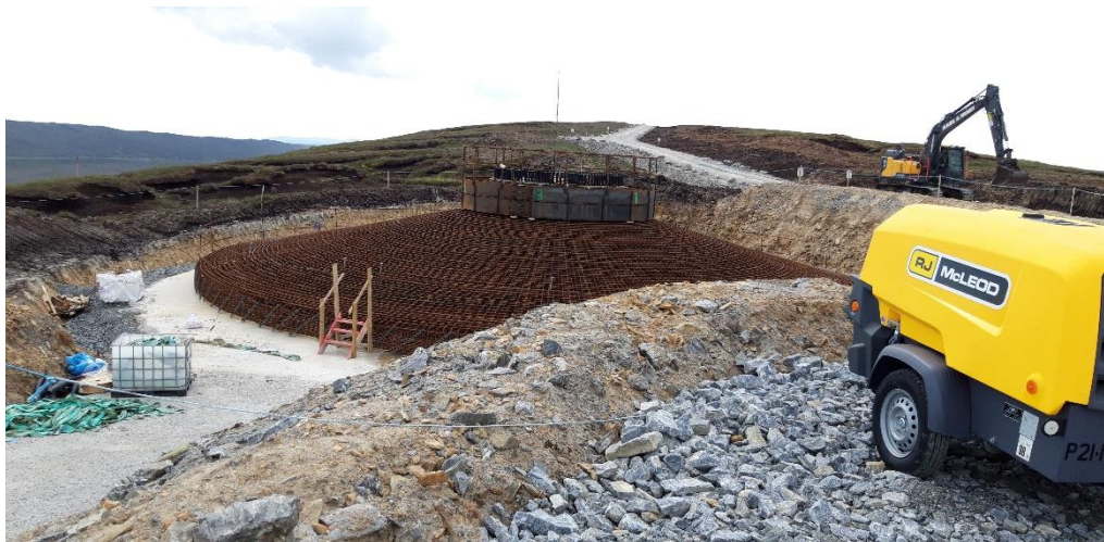
Photo 6. View of the base of K82 which is progressing towards concrete pouring.
