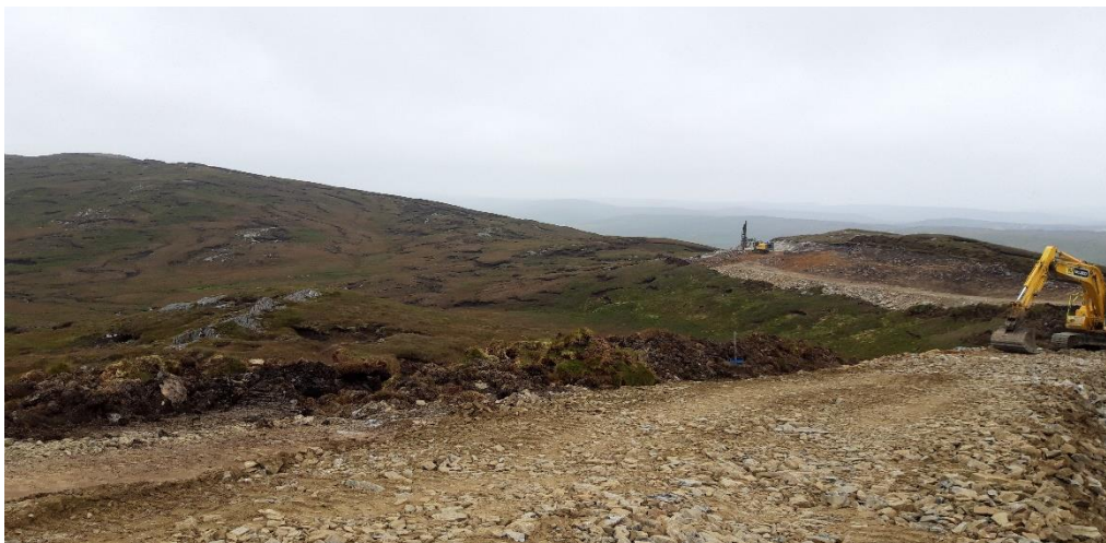
Photo 2. View of peat reinstatement on Spur 14, the peat and turf is built up to the track level as construction progresses.
