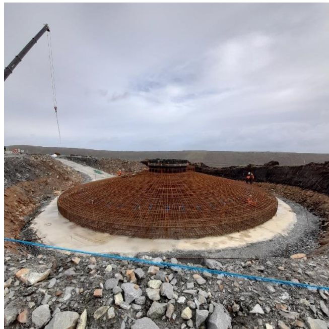
Photo 7. View of the steel work at K86 in preparation for concrete pouring.
