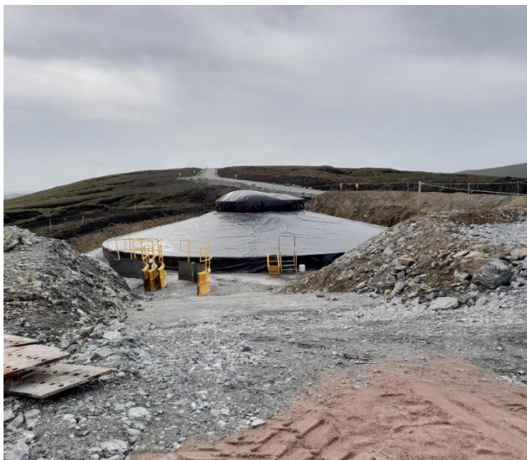
Photo 8. View of the completed and covered concrete work at K82, the excavated area will then be backfilled.
