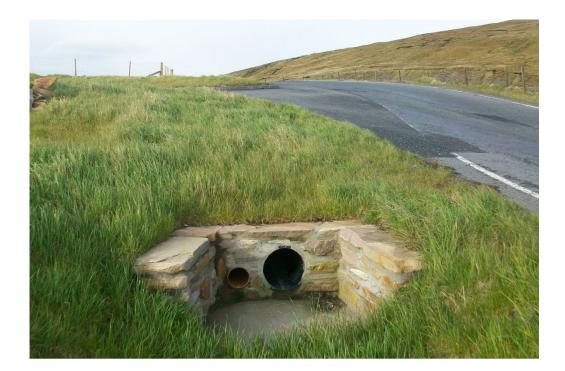
5.2.4 Depending on local conditions the ditch to be crossed may need to be deepened and re-graded to accommodate the required pipe diameter. Where the existing ditch is shallow and/ or close to the existing road it may need to be re-located to ensure that a suitable roadside verge width is maintained. Prospective developers need to ensure that they have access to adequate land to carry out any required alterations to the roadside ditch.
