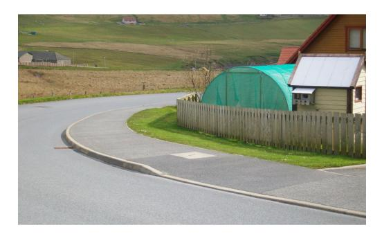
3.5.5 To calculate the clear area of ground required around a bend for forward visibility a line representing the driver's position is drawn 1.5 metres in from the nearside road edge or kerbline. The appropriate forward visibility distance is marked every 10 metres along the driver's path and the end points connected by a chord line. The area within these lines forms the visibility splay area to be kept clear.
