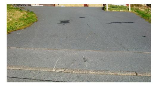
4.5.4 On longer accesses (>50m) vehicle speeds over 20mph are common and so the sharpness of the vertical curve (the K value) should be limited, as should minimum lengths to prevent grounding. On shorter accesses (driveways) only the recommended minimum overall lengths of the vertical curves are noted. The recommended limits are:-
