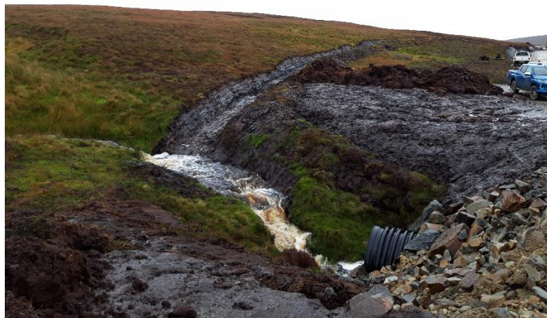
Photo 2. Example of cut off trenches that direct clean surface water flow away from construction areas at K64 (inflow)
