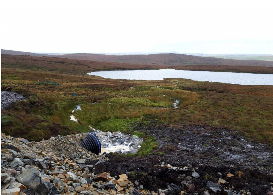
Photo 3. Example of working culvert under track to K64 (outflow)
