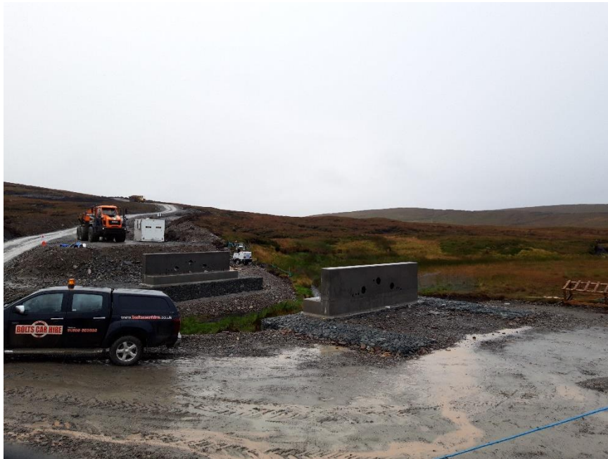
Photo 11. View of completed concrete abutment at watercrossing 19
