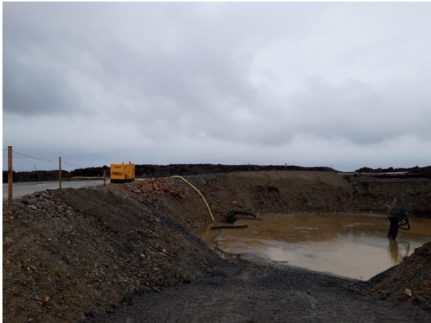
Photo 1. Water pump being used at K47 in preparation for installation of steel cages
