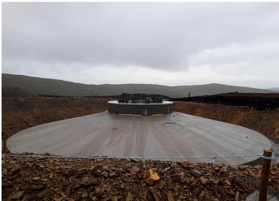
Photo 4. View of exposed concrete work at K79, the excavated area will then be backfilled
