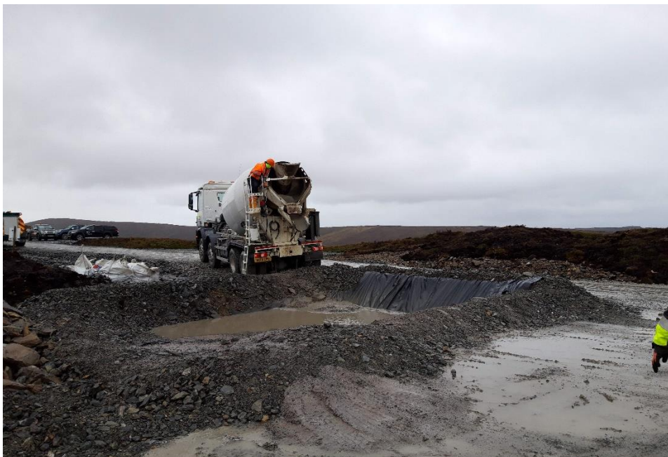
Photo 6. Rinsing of vehicle being used for concrete pouring with mitigation in place to avoid pollution and run offs.
