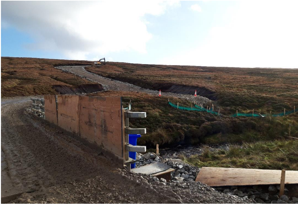
Photo 7. Splash guards installed on temporary bridge at watercrossing 15 and view towards tracks onto N96
