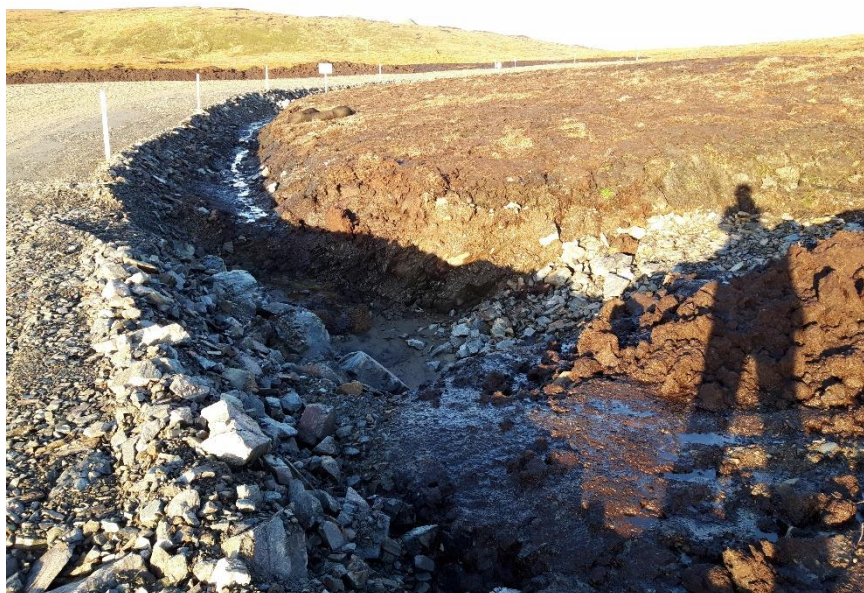
Photo 10. Example of dirty water system near N132
