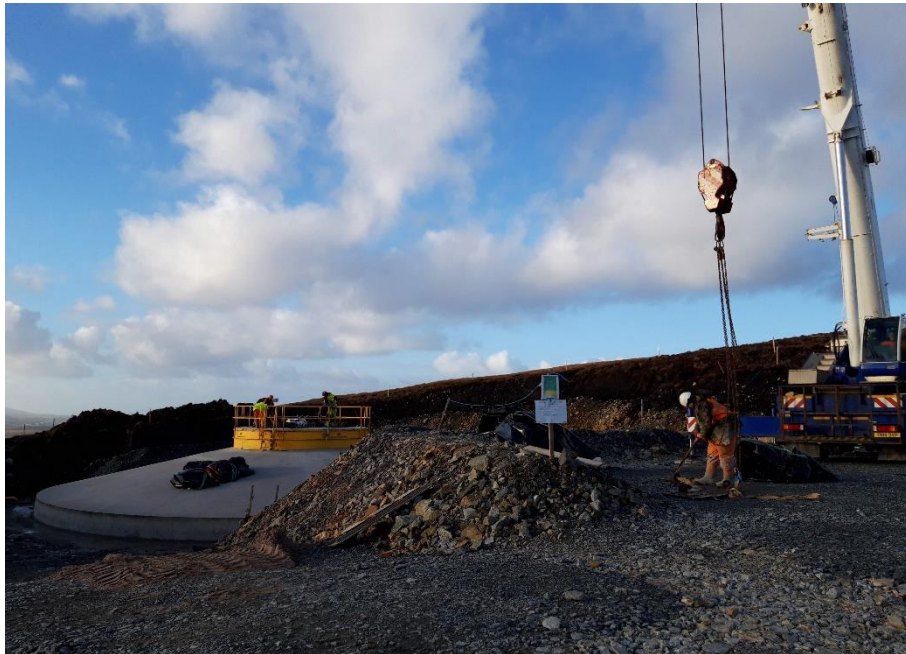
Photo 3. Shuttering being lifted at K48 after concrete pour
