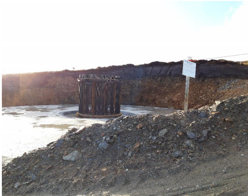
Photo 2. Example installed central pillar over concrete blinding at K44, before steel fixing
