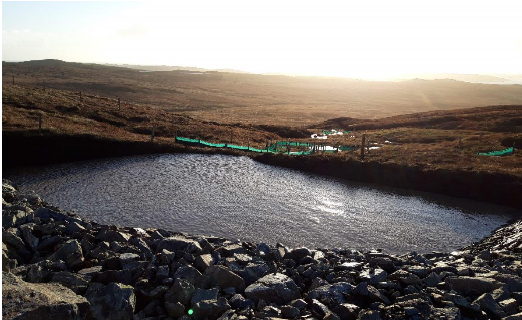
Photo 11. Example of track side settlement pond near N132
