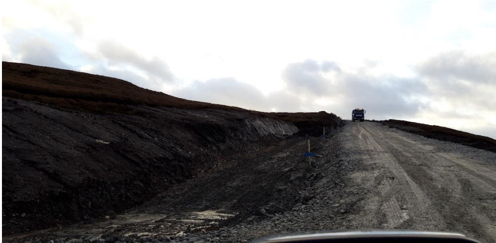
Photo 5. View of the excavation in preparation for cables to be installed on Mid Kame Ridge.
