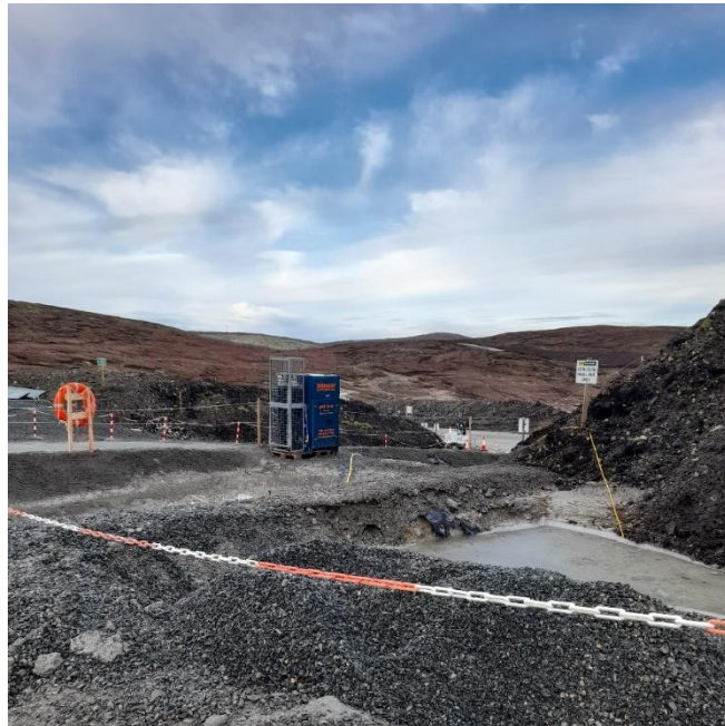
Photo 7. Concrete washout at batching plant
