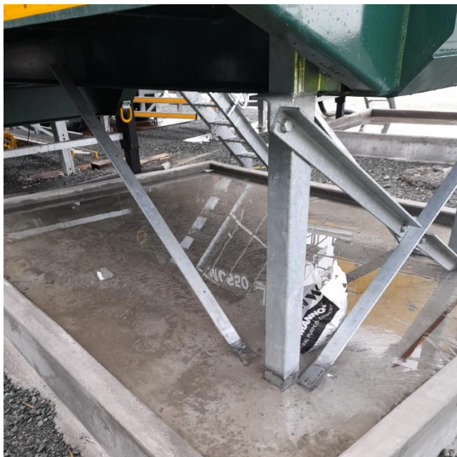
Photo 10. Rainwater accumulation in bund
