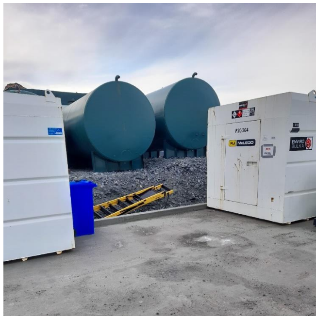
Photo 8. Batching plant fuel storage and spill kit
