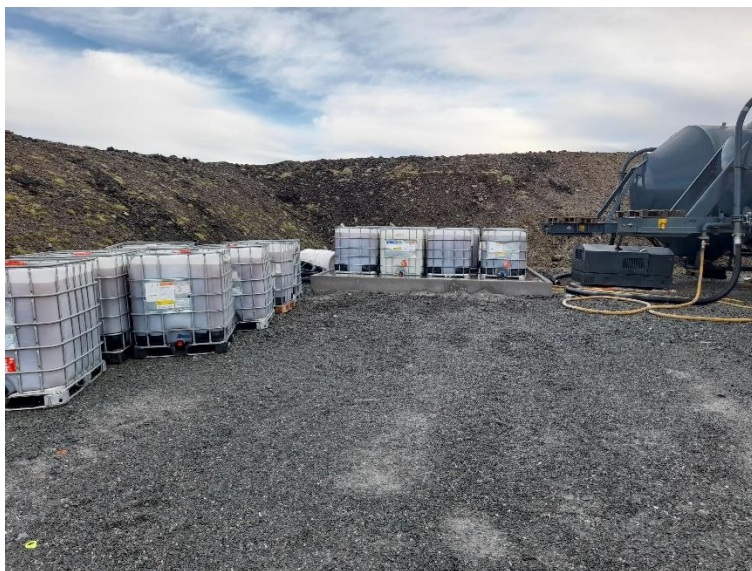
Photo 6. IBCs with concrete admix exceed capacity of storage area
