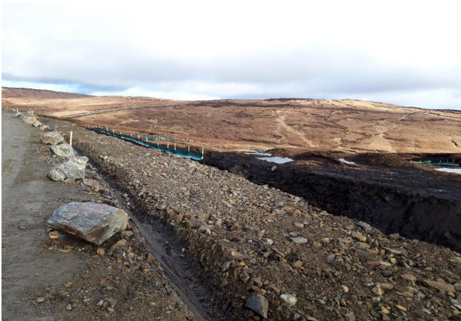
Photo 8. Completed cable trench preparation near N119 awaiting cable laying activities
