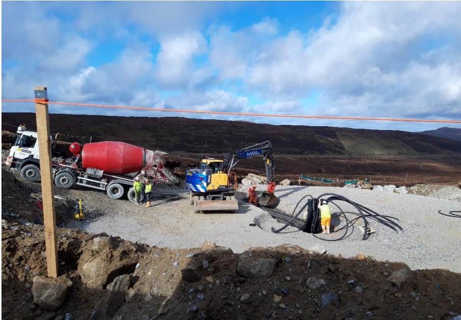
Photo 5. N90 duct trench construction in progress
