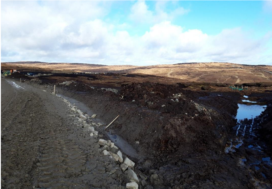
Photo 9. View of drainage by cable trench at Junction 27
