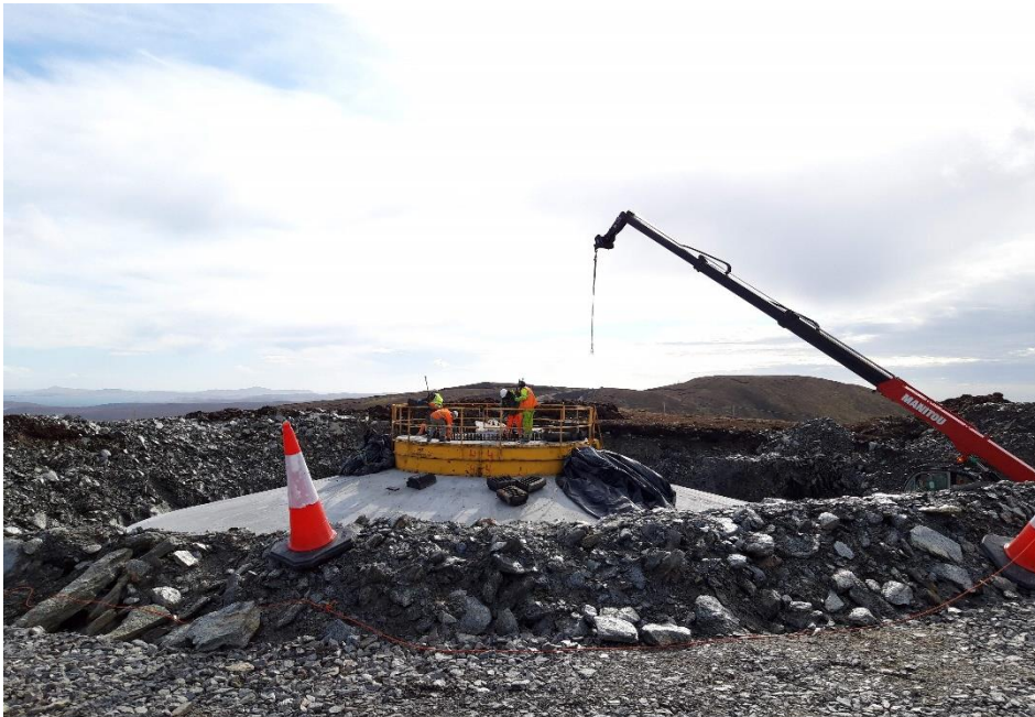
Photo 2. K45 turbine base shutter removal in progress
