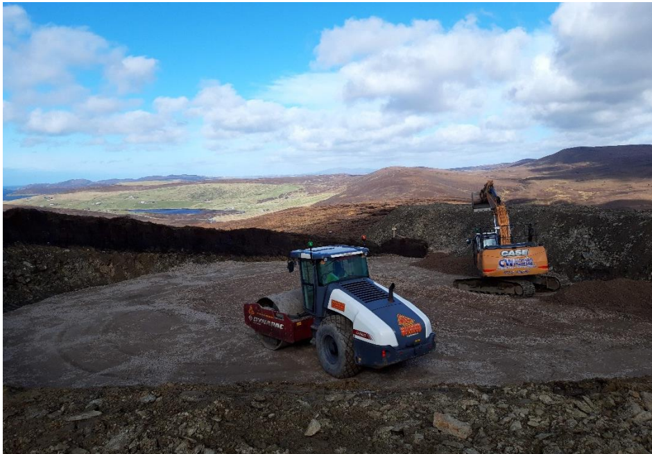
Photo 1. K71 turbine base excavation in progress
