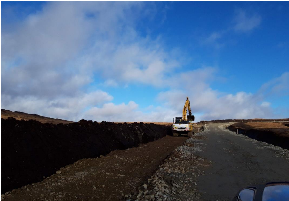
Photo 7. Cable Trench Excavation in progress near N132
