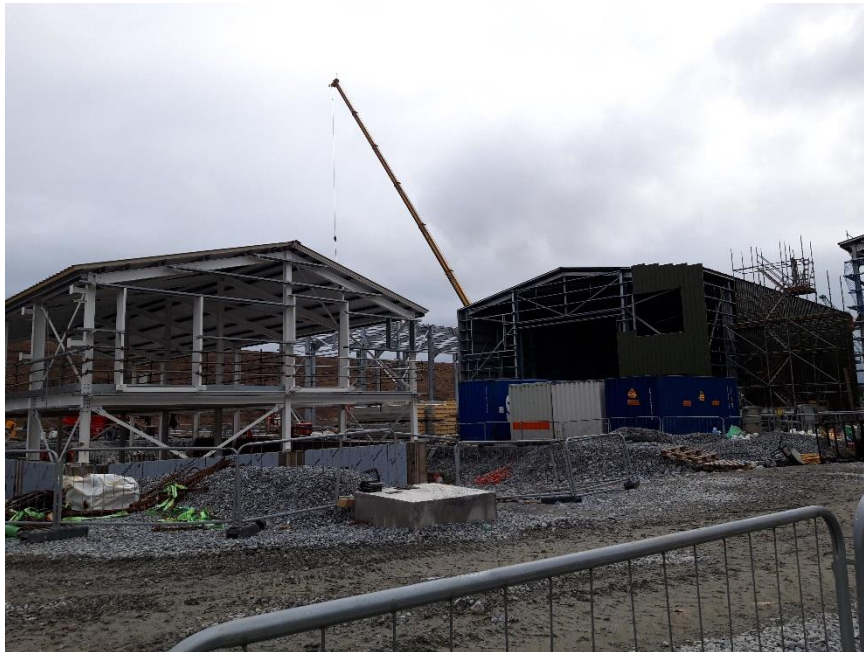
Photo 13. Completed roof cladding on two of the buildings in the substation area
