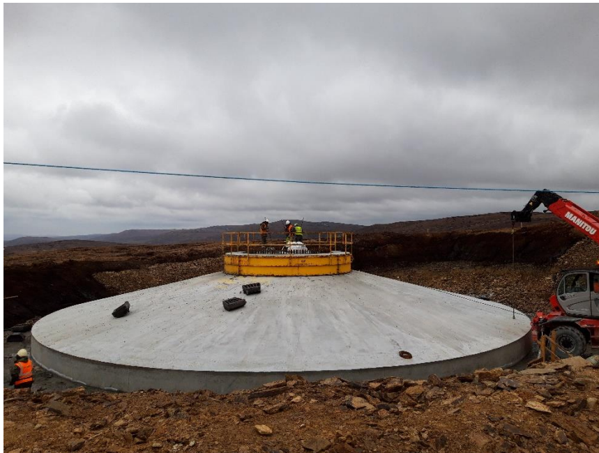
Photo 3. View of shutter removal in progress at K75
