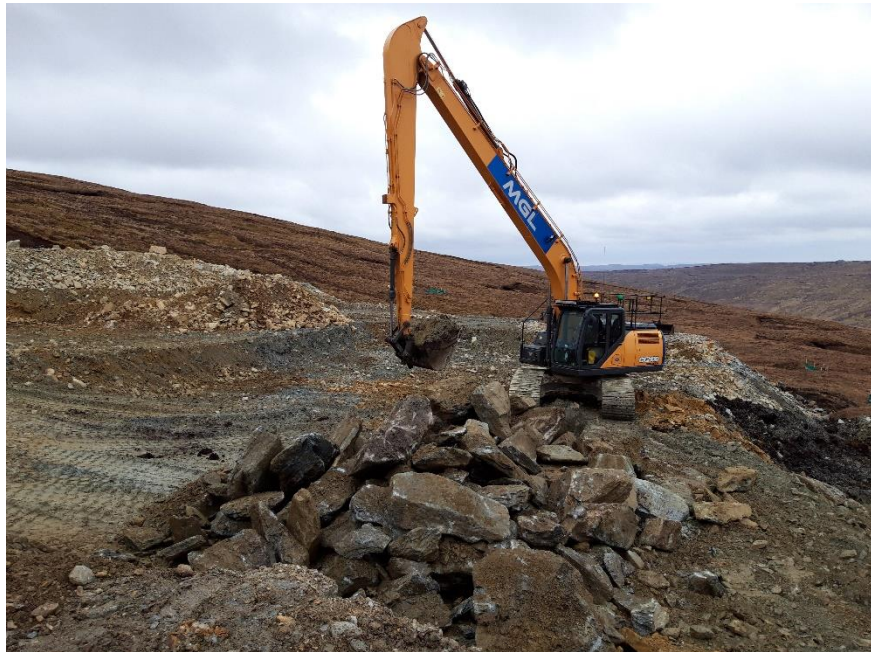
Photo 1. Additional bund support between K51 blade fingers.
