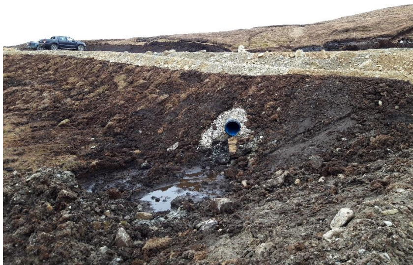
Photo 2. Additional culvert installed at K51
