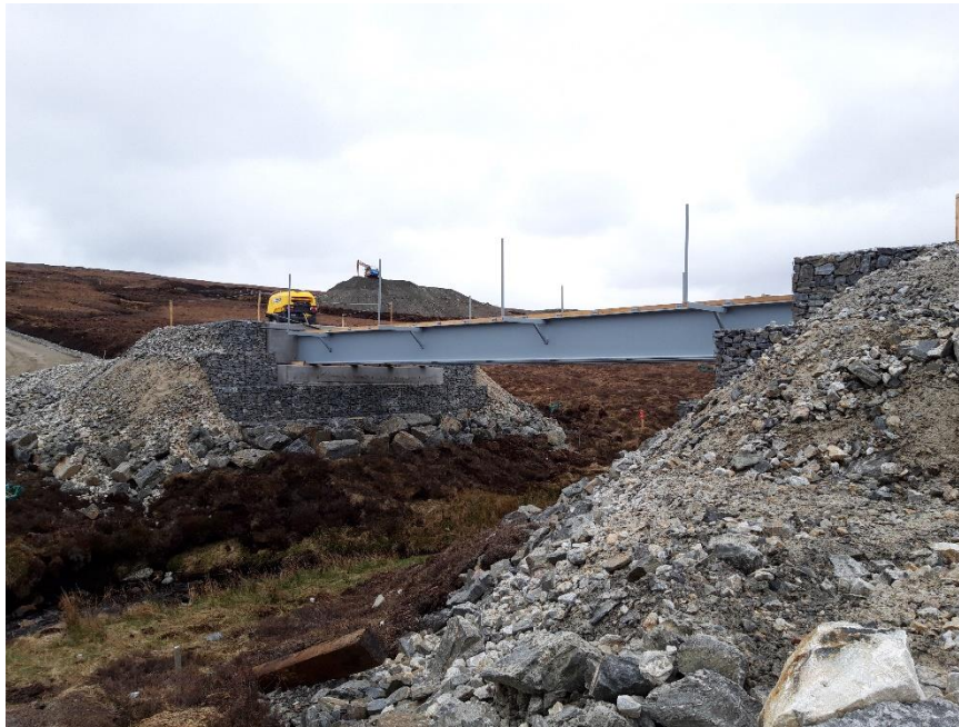
Photo 7. Permanent bridge steel base installation at WC15
