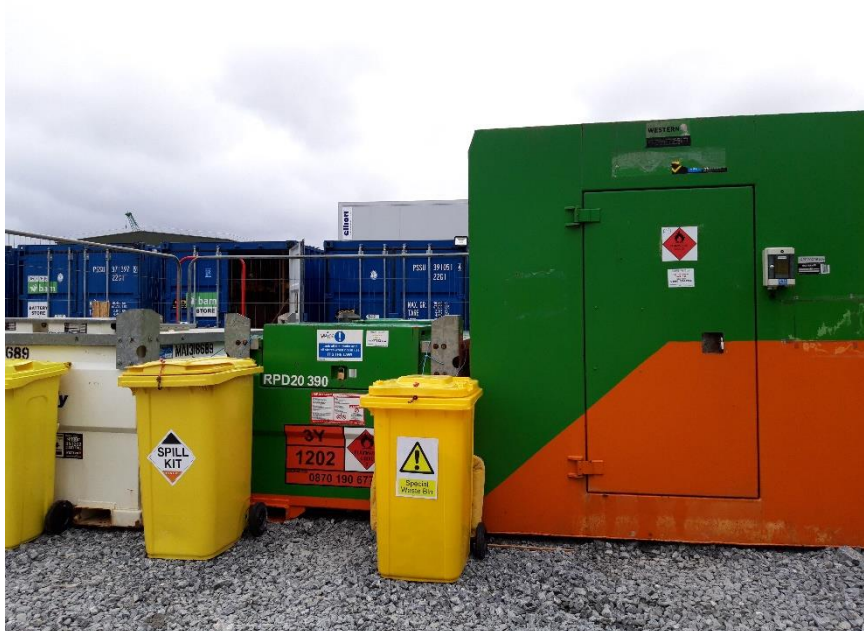
Photo 14. Fuel storage at substation with spill kit
