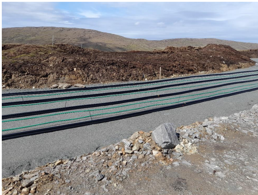
Photo 6. Cables being laid in cable trench at Mid Kames Ridge.
