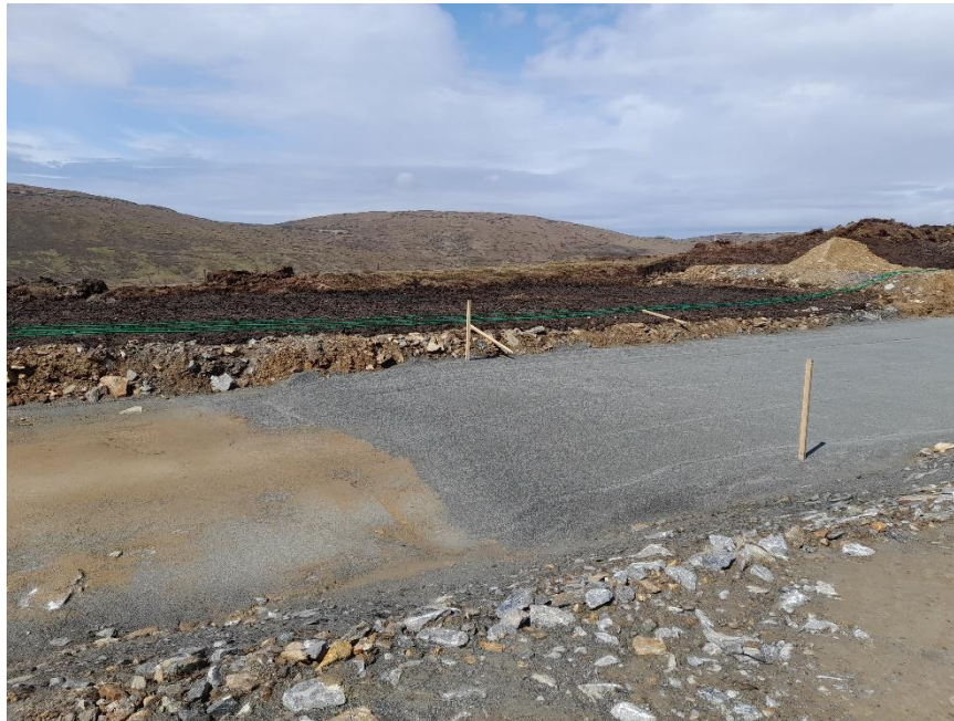
Photo 5. 75 m of "Whin-Dust" being laid as cable bedding.
