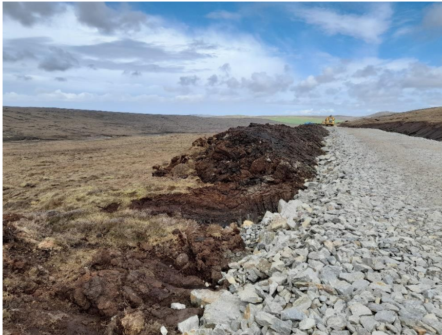
Photo 3. Good segregation of turf and peat at the track at Spur 6, towards K68.
