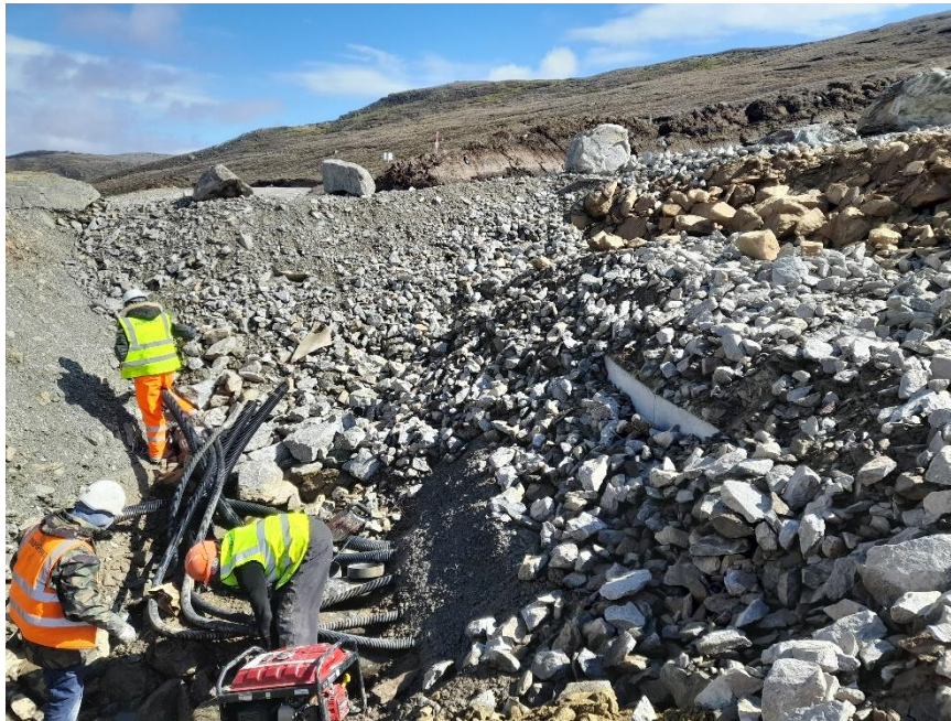
Photo 1. Backfill of base, and cable ducting at K62.
