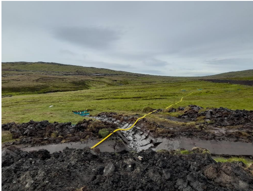
Photo 11. Longer hose route for water being pumped from base
