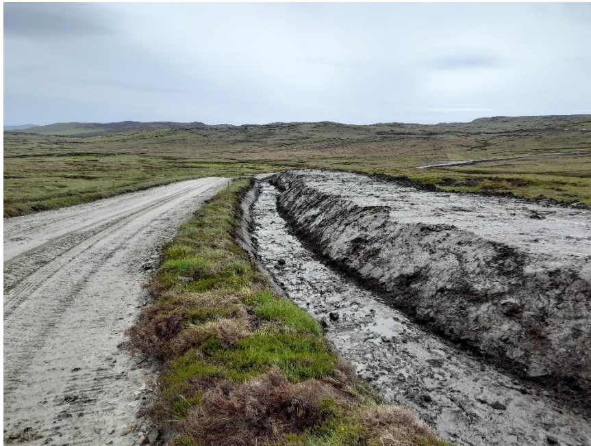
Photo 9. Cable trenching works between N140 and N141
