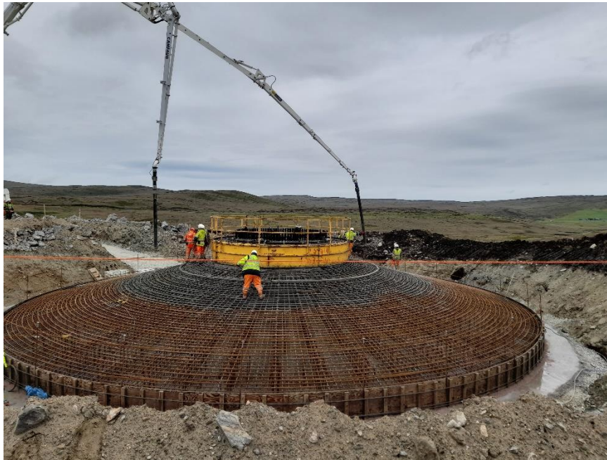
Photo 5. N95 base being poured
