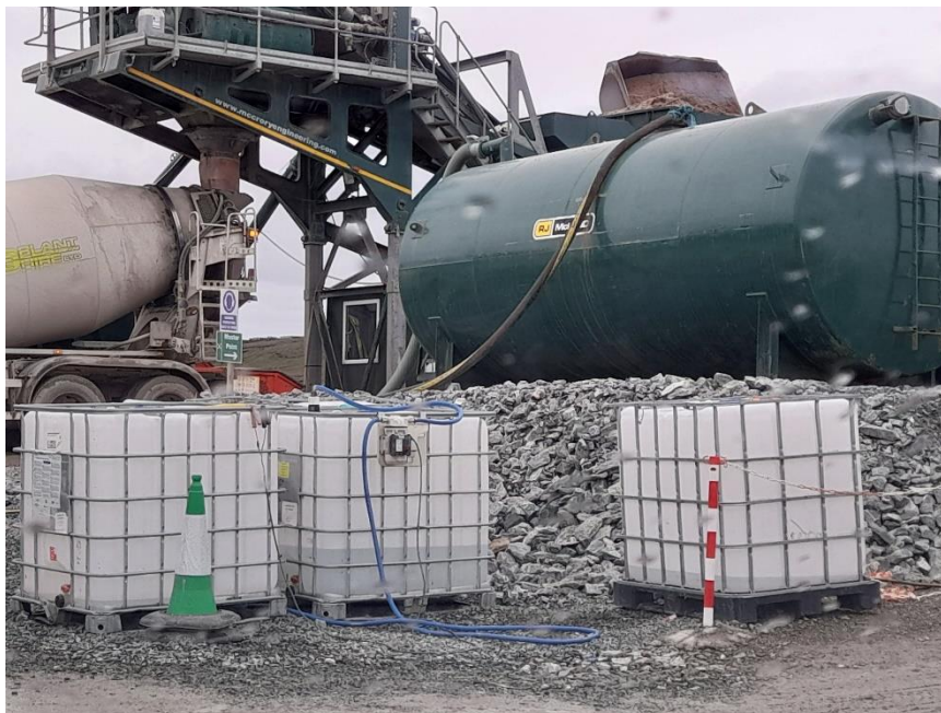
Photo 4. IBCs directly on compacted stone surface
