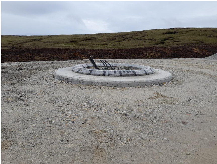
Photo 7. N89 base backfilled
