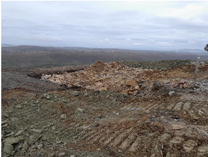
Photo 1. Toe bund between blade fingers at K44
