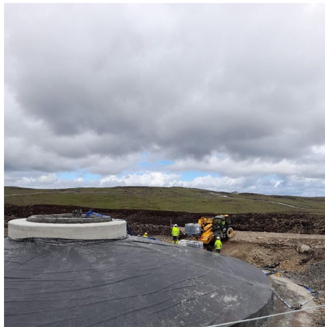
Photo 14 N119 – curing using recirculated water
