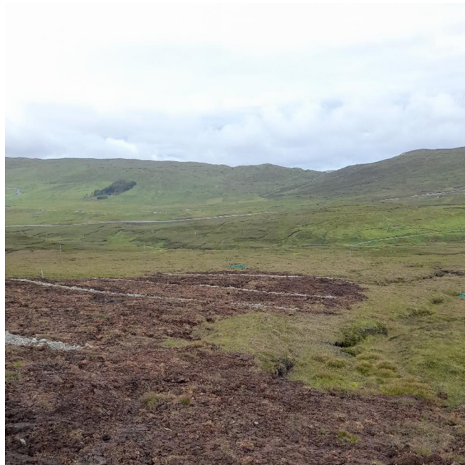
Photo 9. Peat Landslide on west side of MKR following reinstatement
