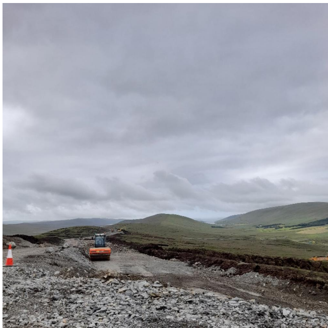
Photo 8. MKR Cable Track/Trench Preparation
