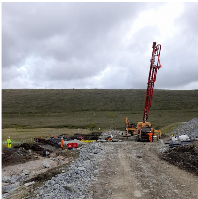
Photo 16 Cable ducting works under the substation perimeter drain
