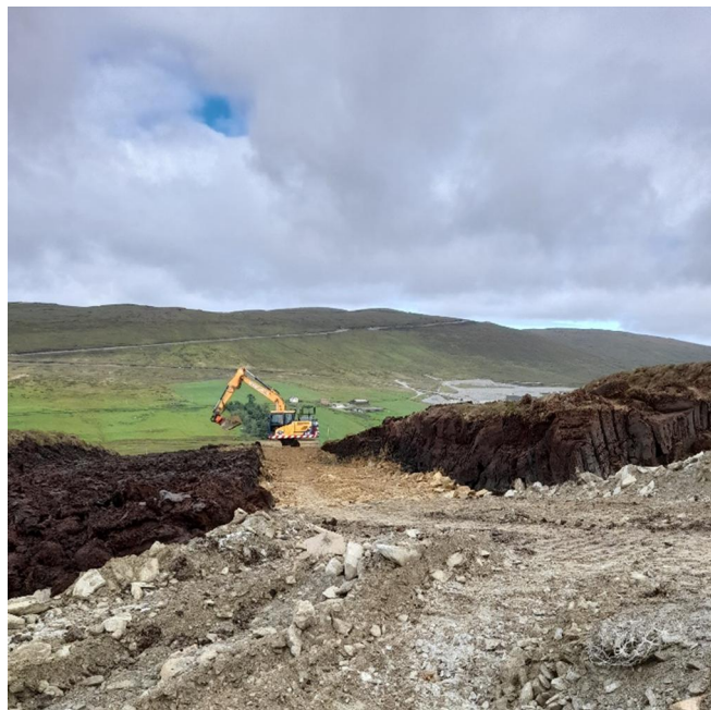
Photo 10. Start of temporary track construction for cross country cable to connect to substation from MKR
