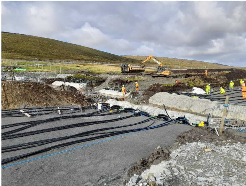
Photo 13. Construction of substation cable under previous location of Northern Watercourse
