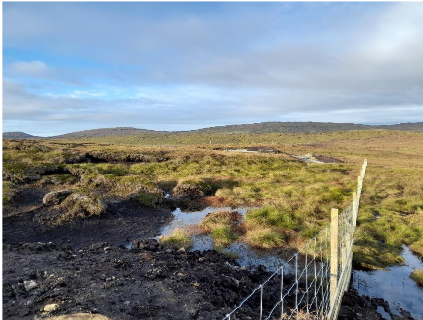
Photo 11. Fencing installed at P11 peat restoration area
