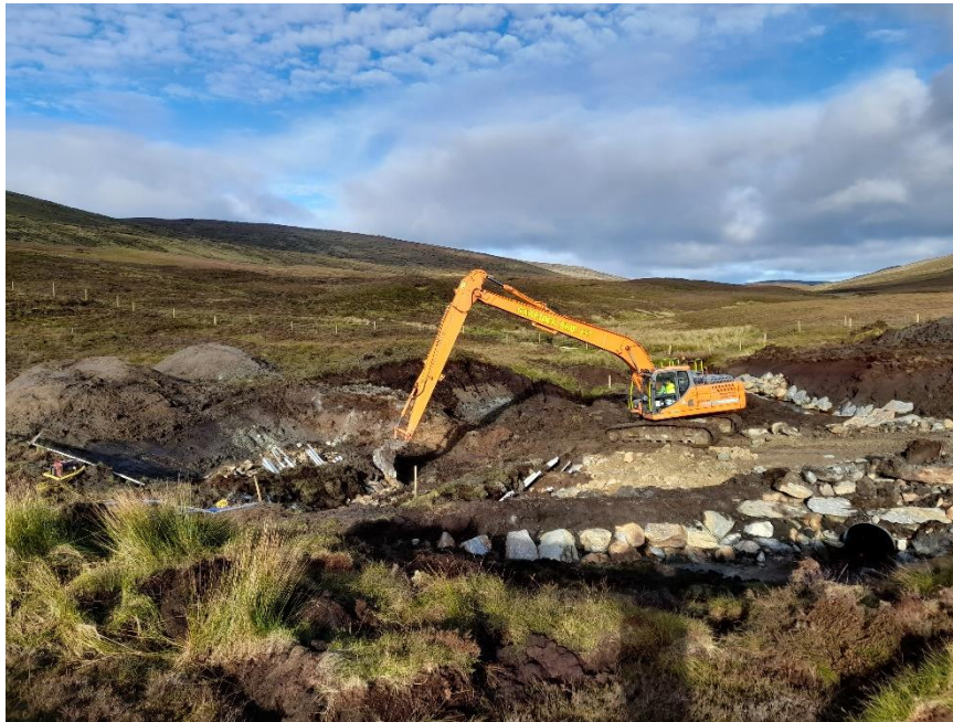
Photo 5. Burn of Weisdale Diversion
