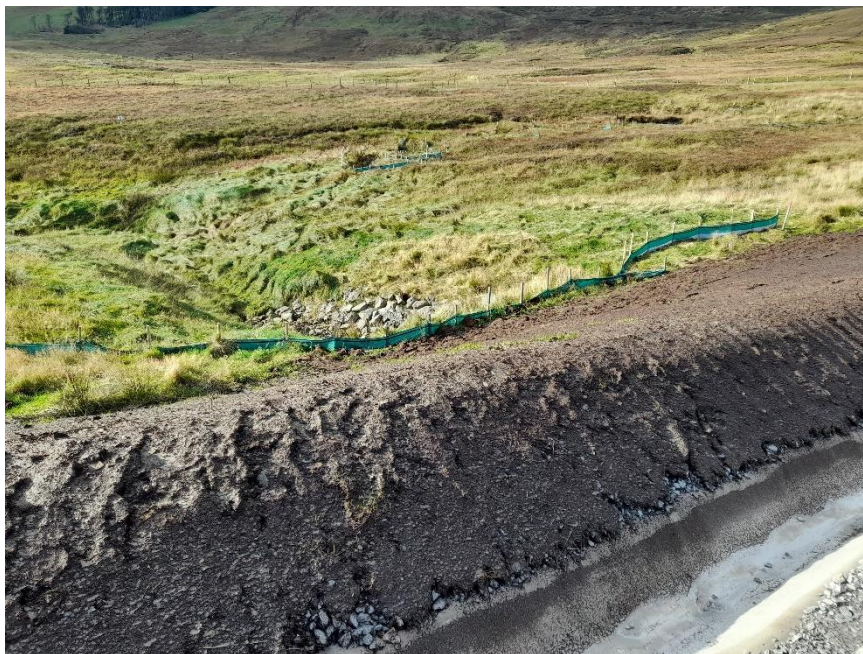
Photo 2. Surface water drainage at the Droswell Burn
