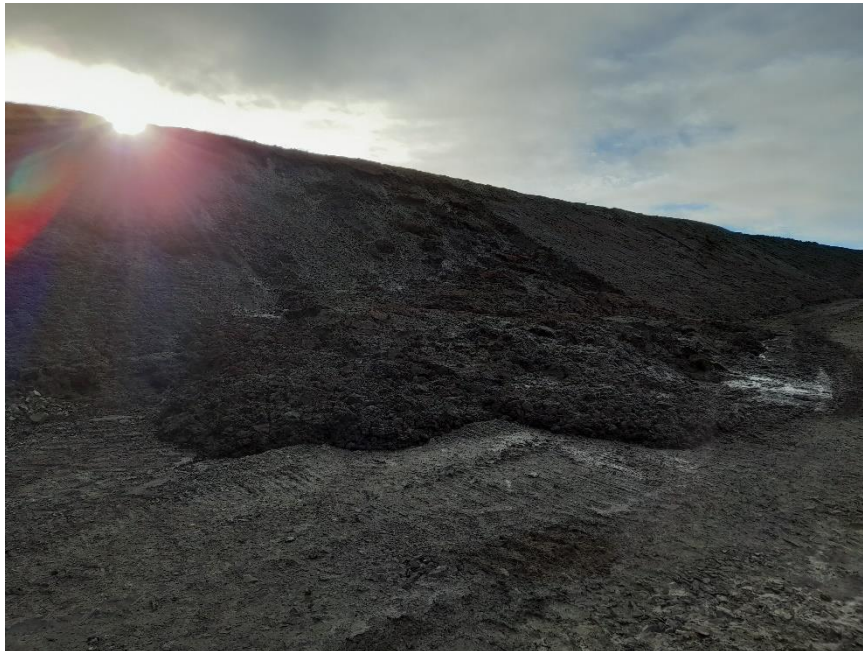
Photo 12. Peat movement in cutting in Spur 52
