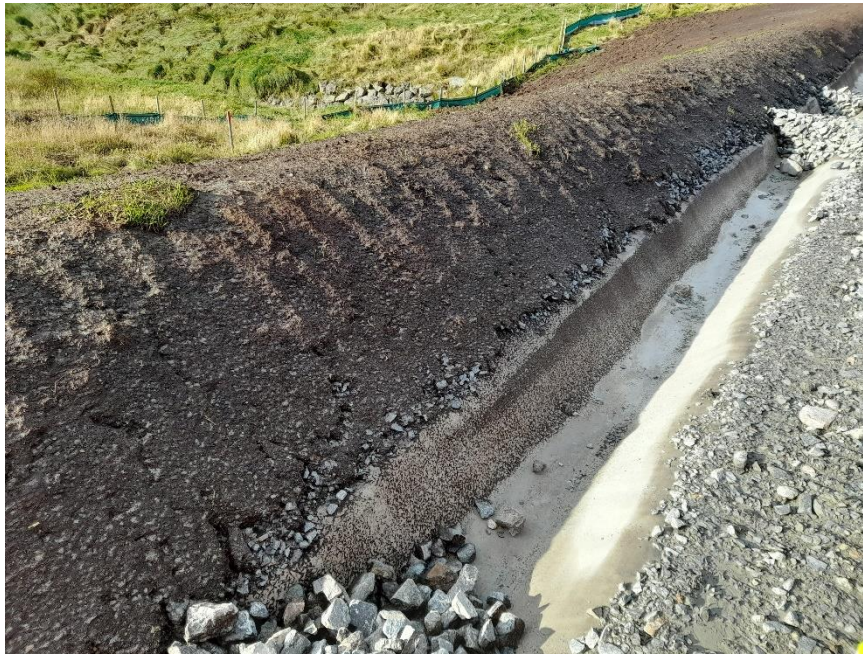
Photo 3. Surface water drainage at the Droswell Burn
