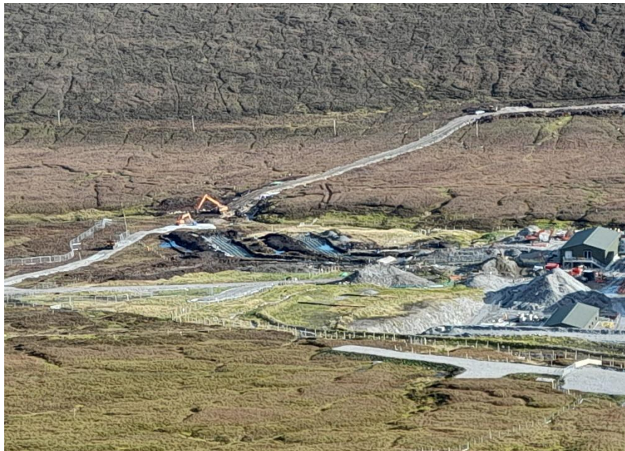
Photo 17. Laying of cable from Burn of Weisdale to substation
