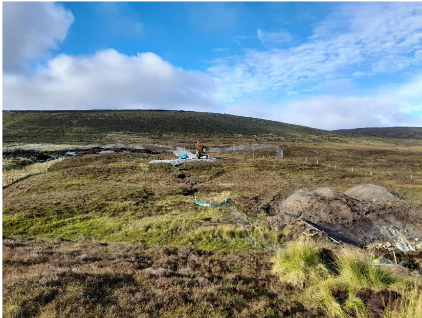
Photo 16. Laying of cable from Burn of Weisdale to substation
