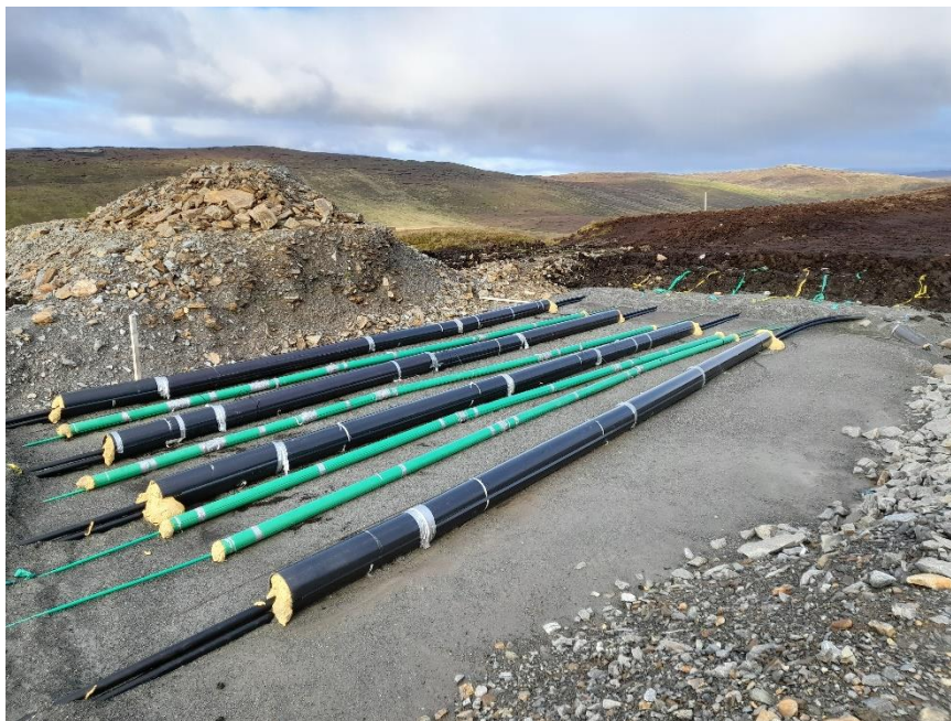
Photo 4. Cable trenches awaiting backfilling on Mid Kame Ridge
