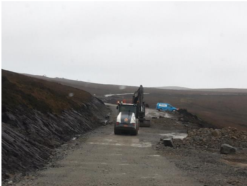
Photo 3. Widening track between K61 and K62
