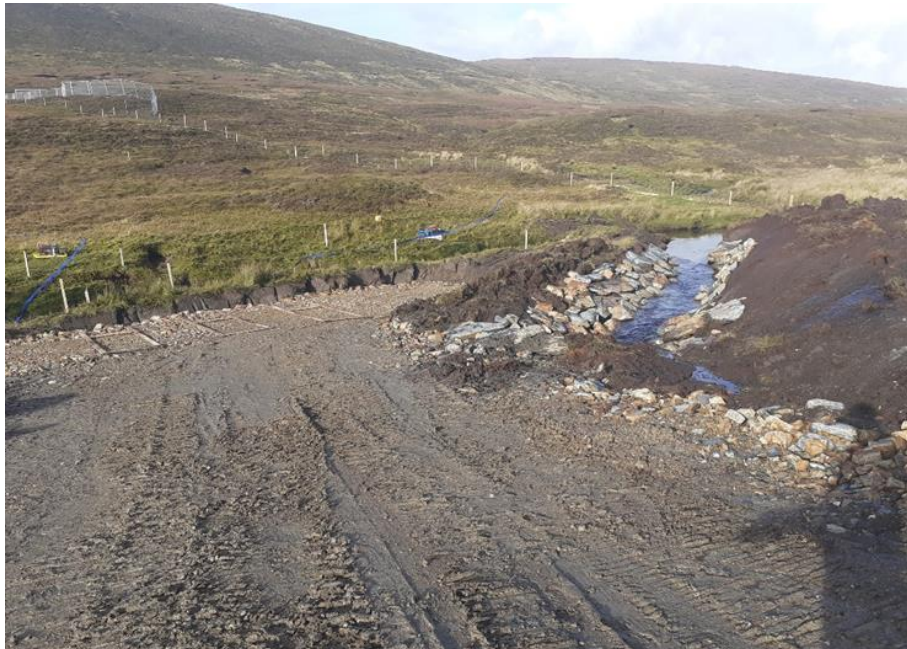
Photo 6. Ongoing Burn of Weisdale diversion (Photo from RJ McLEOD)
