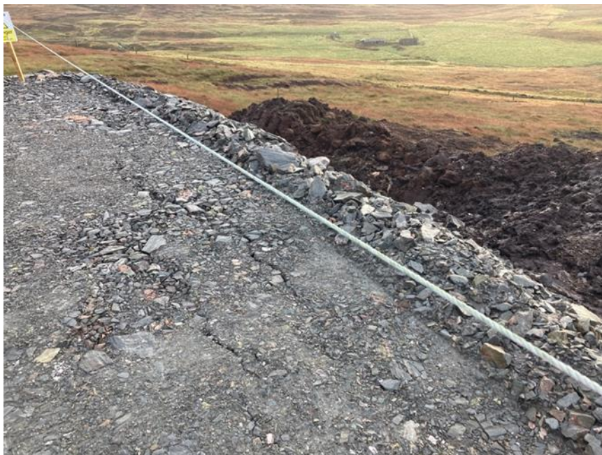
Photo 14. Noted cracks at Turbine Hardstanding N114 currently under investigation (Photo from GCoW)
