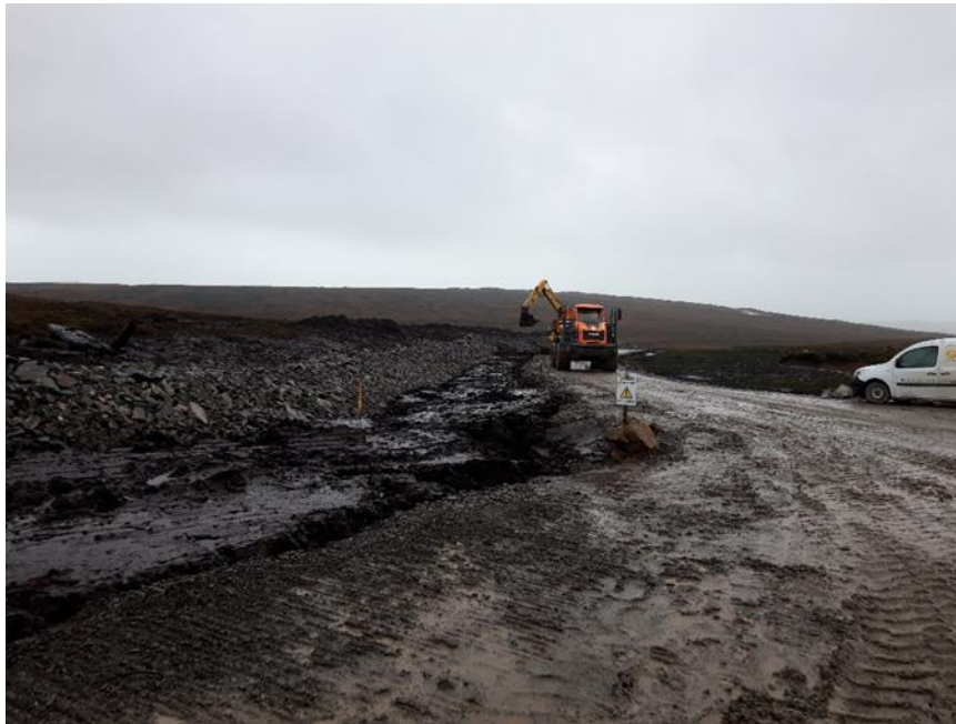
Photo 13. Cable trench near N118 being backfilled
