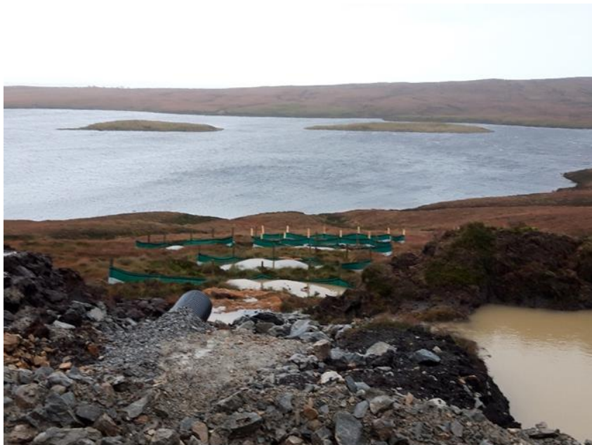
Photo 2. View of drainage system near Maa Water: Settlement pond, culvert and silt traps
