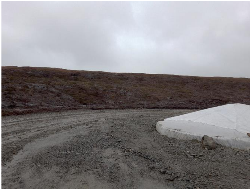
Photo 9. N96 turbine base backfilled, drainage amended and prepared for turbine erection activities
