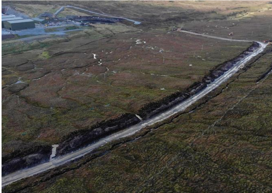
Photo 5. Aerial view of cross-country cable route into substation with drainage and other mitigation (Photo from RJ McLEOD)
