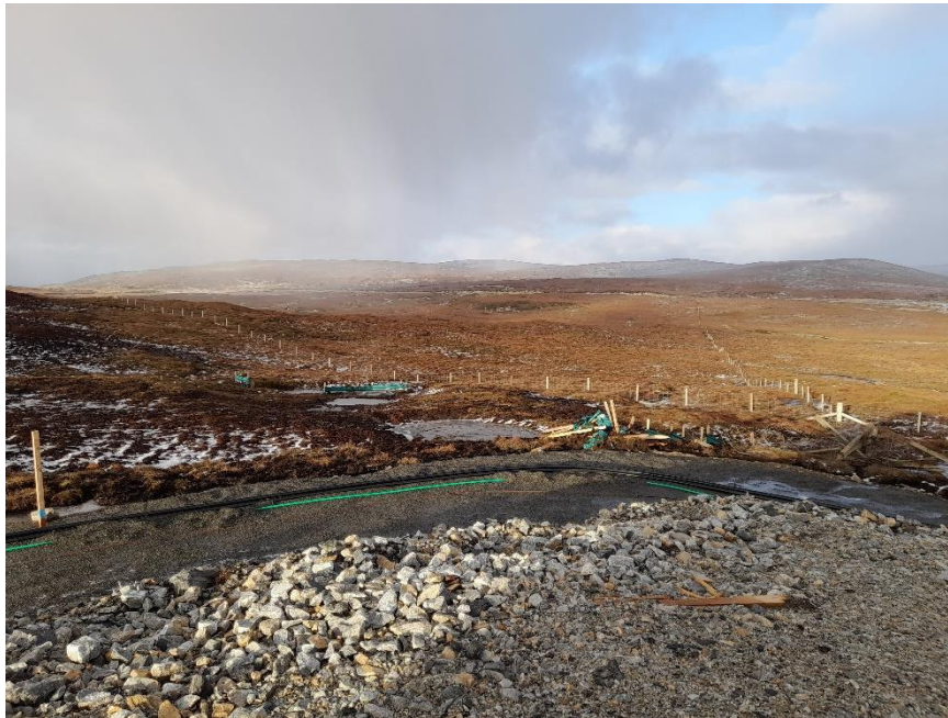
Photo 9. Silt fences have been maintained and settlement ponds installed for longer term drainage solutions between N92 and N95.
