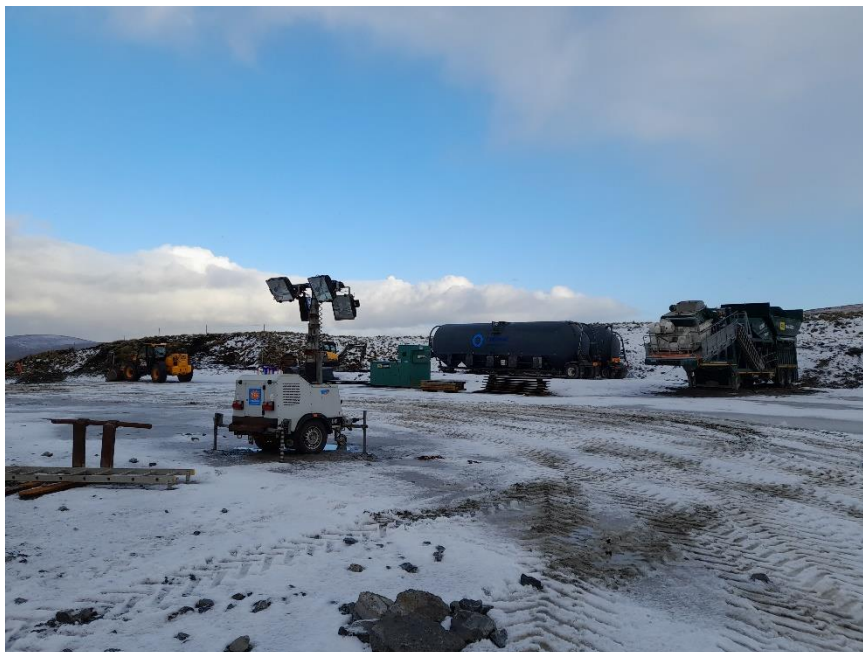
Photo 6. Removal of tanks from the batching plant in the northern compound
