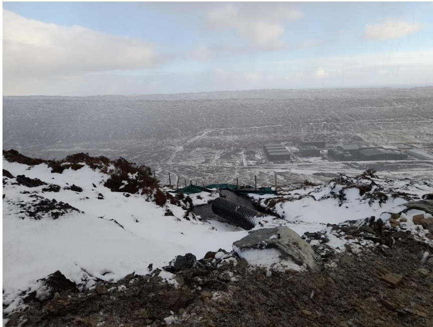
Photo 5. Clean water culverts being installed as the cross-country cable track is progressed from Kergord to the substation
