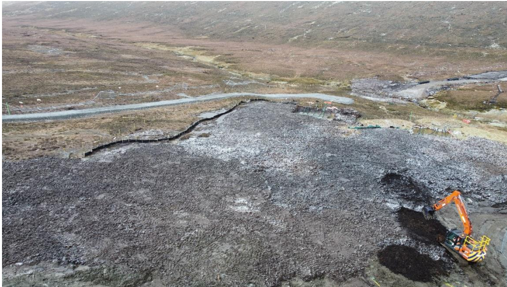
Photo 13. Area around backfilled cables at northern watercourse being relandscaped (Photo courtesy of SSE).
