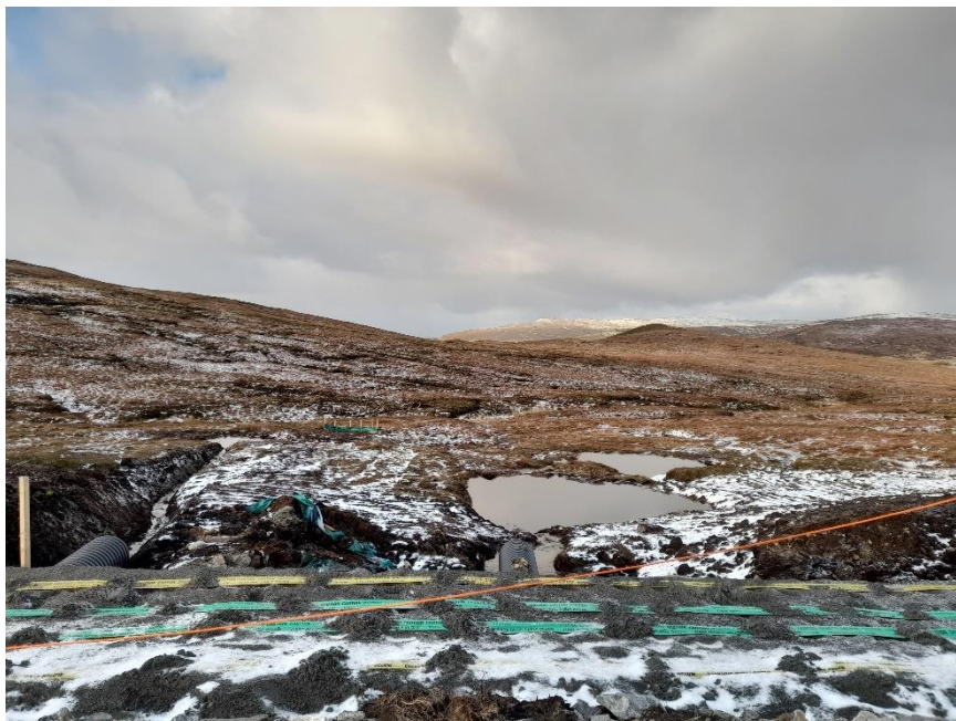
Photo 8. Silt fences have been maintained and settlement ponds installed for longer term drainage solutions between N92 and N95.
