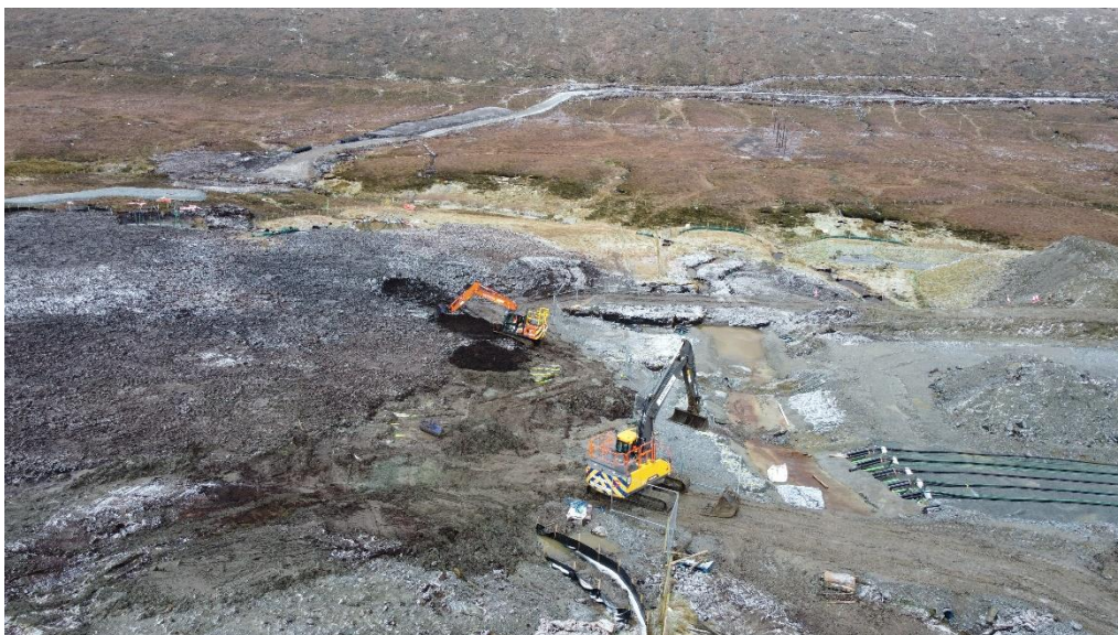
Photo 12. Cable trenches around northern watercourse have been backfilled (Photo courtesy of SSE)
