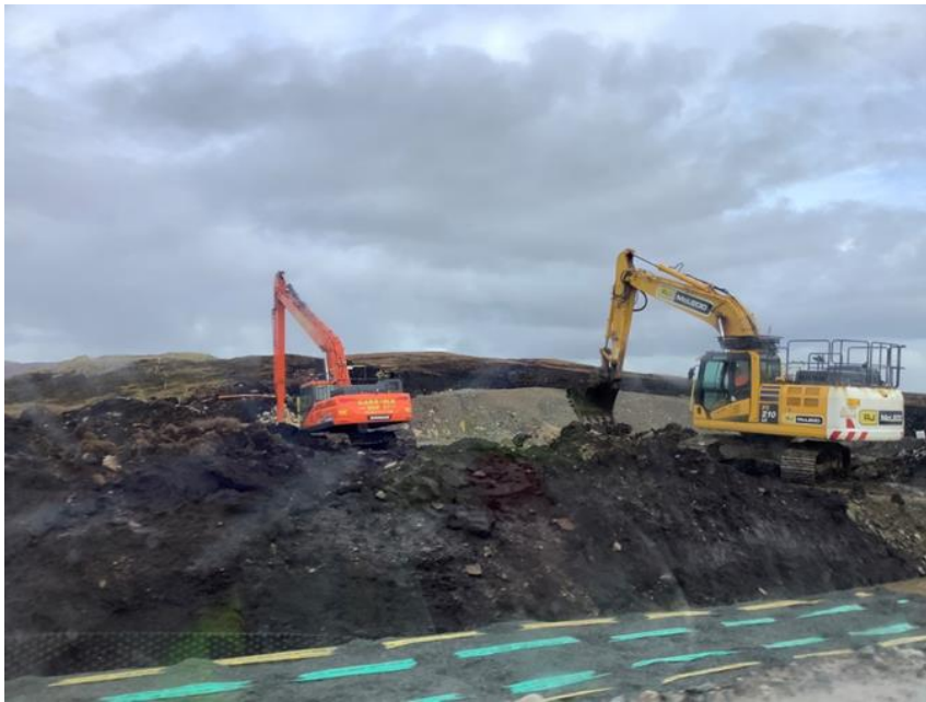
Photo 7. Preparation for backfilling of cable trenches near turbine 048 (previously N90)
