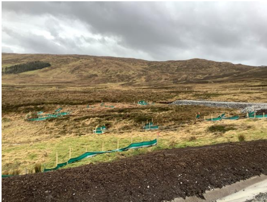
Photo 3. View of silt fences by Droswell Burn
