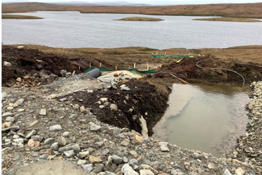
Photo 2. Mitigation by Maa Water with settlement pond, water pump and silt fences
