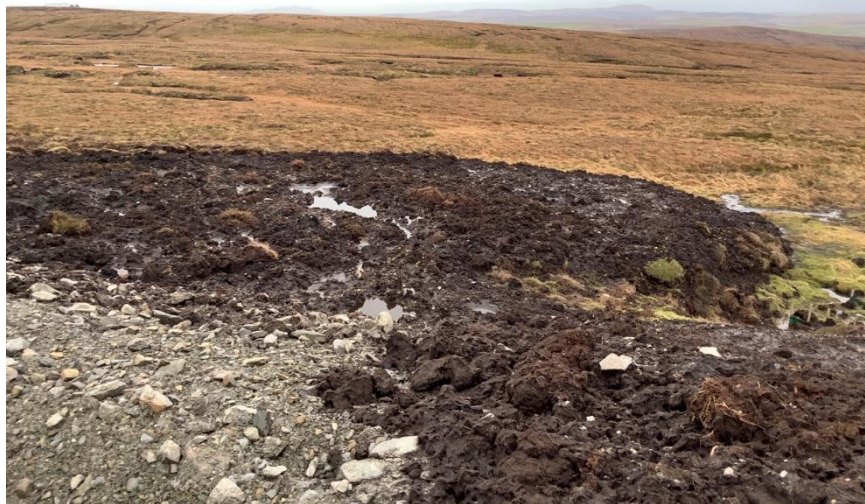
Photo 17. Peat slump at turbine 005 (previously K73)
