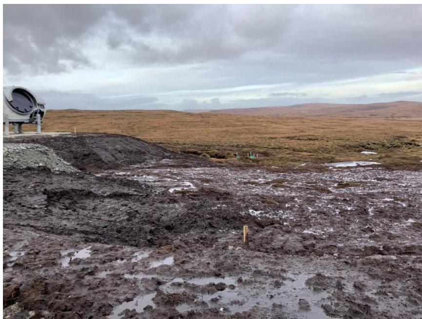
Photo 18. View of turf bund and silt fences for peat movement by turbine 055 (previously N97)
