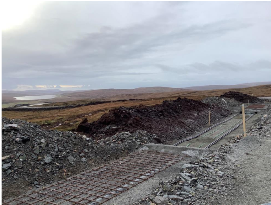
Photo 11. Concrete Protection detail for cables that pass through assist crane hardstands at turbine 073 (previously N114)
