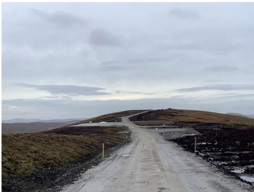
Photo 4. View towards turbine 042 (previously K82) showing capped road and turbine hardstand
