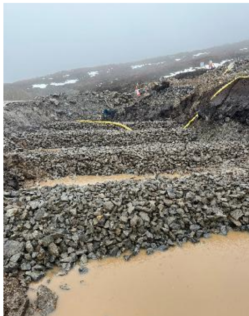
Photo 2. Mitigation by Maa Water with settlement pond, water pump (and silt fences out of shot), by KBP03
