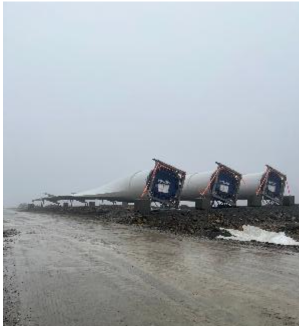
Photo 11. N100 blade laydown on blade fingers
