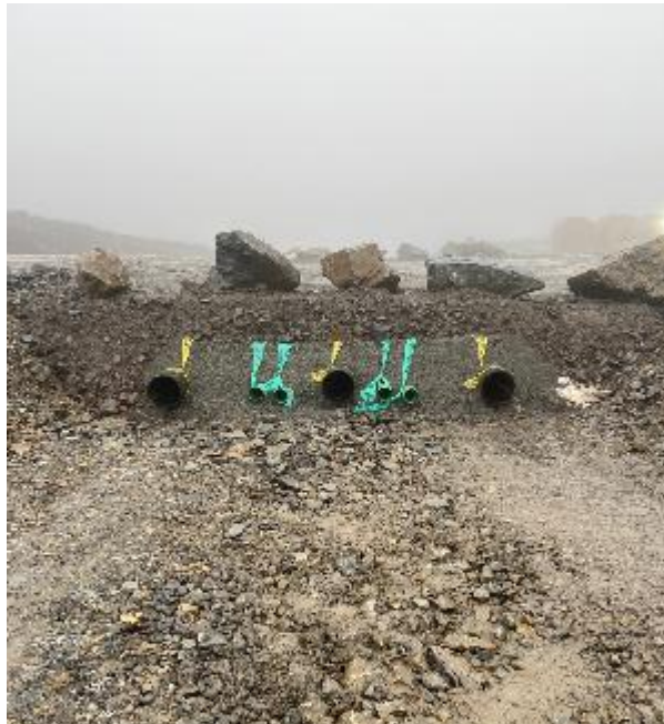
Photo 5. Cable ducts and reinforcement at entrance to Vestas compound (KBP06)
