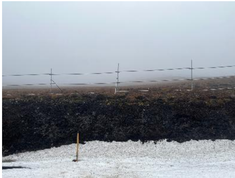
Photo 15. N100 bird mitigation (netting still to be installed on scaffold)
