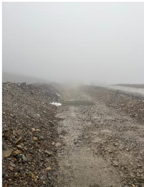
Photo 6. Cable track concrete plug (partially poured)
