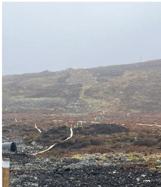
Photo 10. Silt fencing and stone stockpiles adjacent to Sandwater track ready for cross-country cable route
