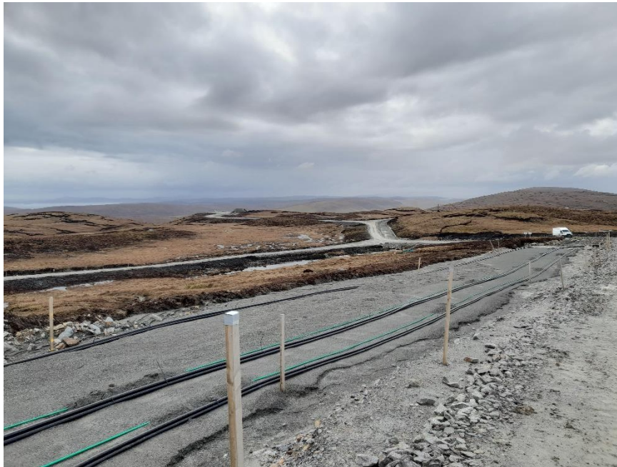
Photo 3. Erosion of cable bedding material
