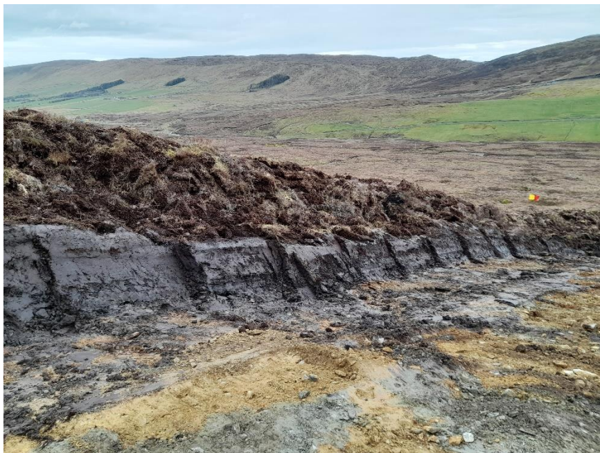
Photo 10. Turf stripping at cross-country cable route
