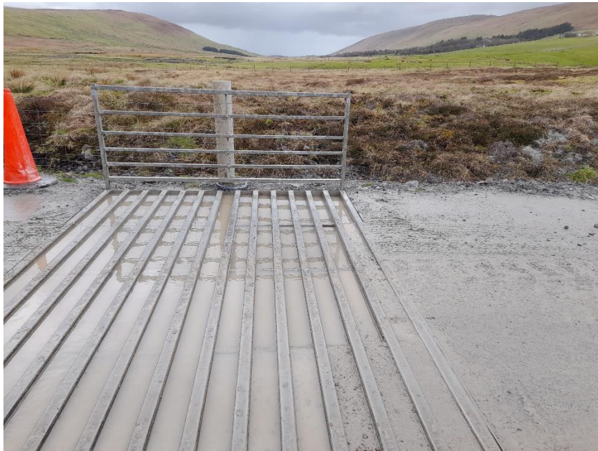
Photo 14. Drainage defects near the Weisdale Burn
