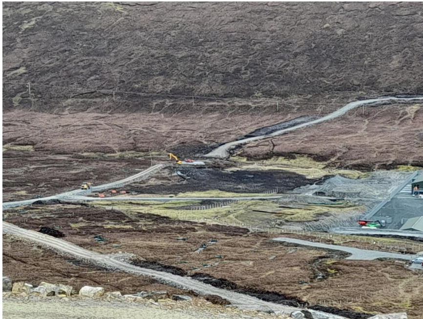
Photo 9. Construction of cross-country cable access track
