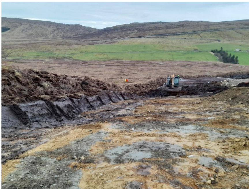
Photo 11. Cable trench excavation at cross-country cable route
