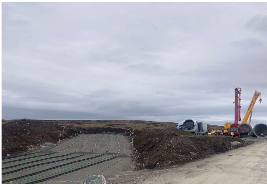
Photo 12. Cabling trench and cranes at T069
