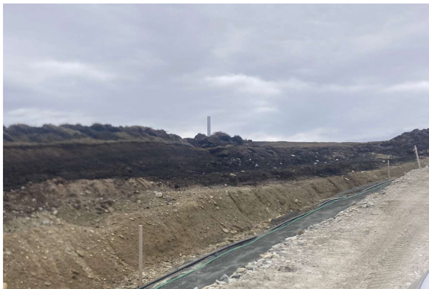
Photo 10. Cable trench requiring backfilling north of T047
