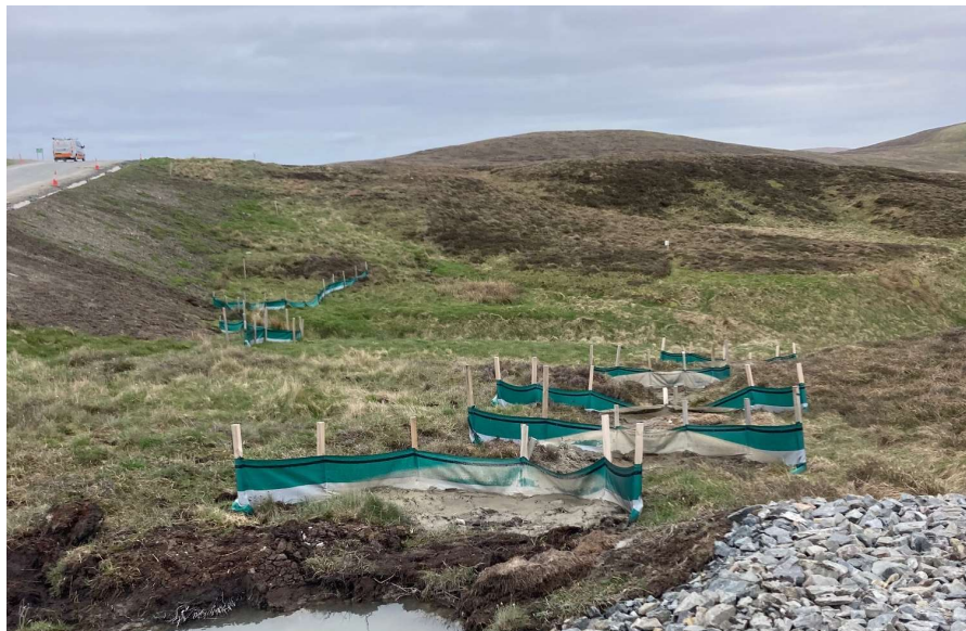
Photo 5. Silt fences at the Droswell Burn
