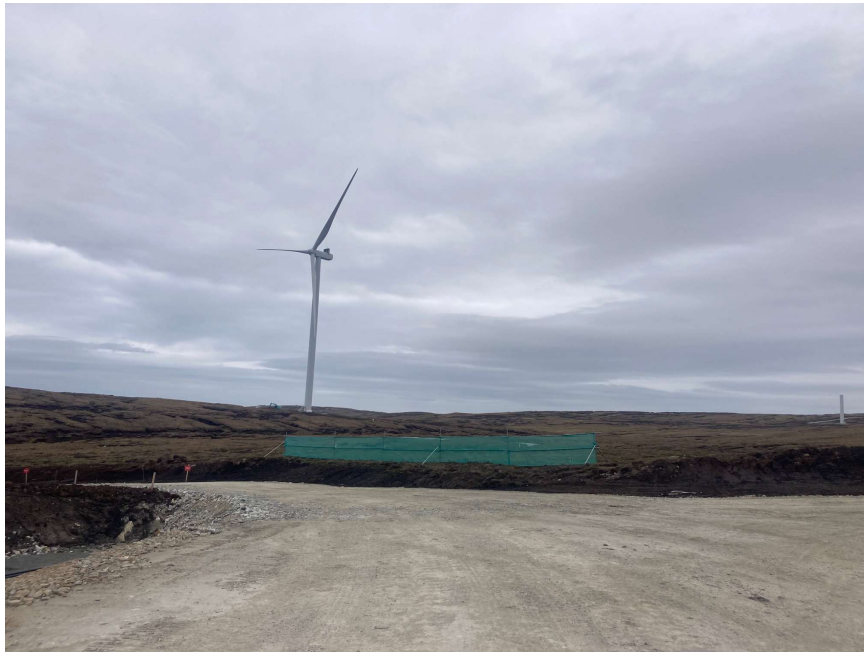
Photo 11. Screen at T058 to limit visual disturbance to nesting birds
