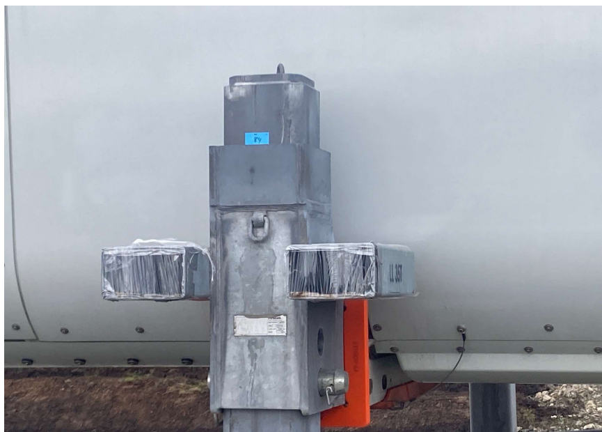
Photo 14. Plastic wrapping covering supporting frame hole at T075 as bird deterrents
