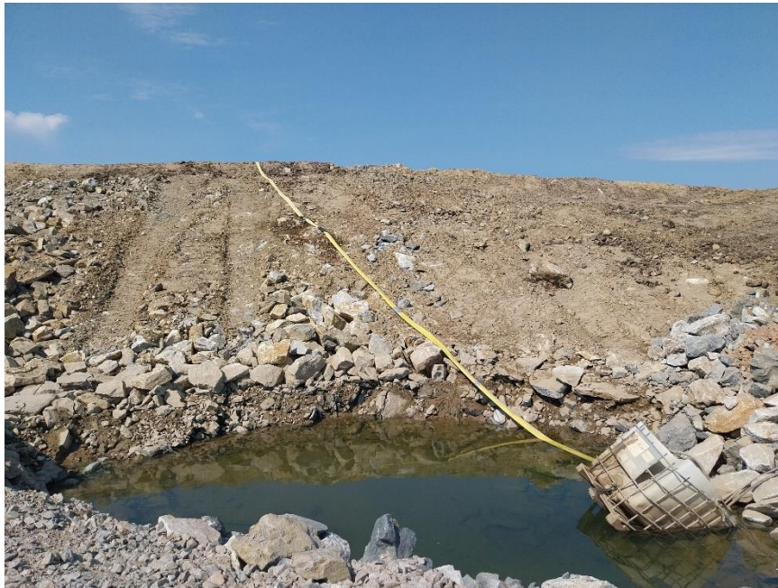
Photo 11. Settlement pond utilised to supply water to bowzers for dust suppression management at NBP01
