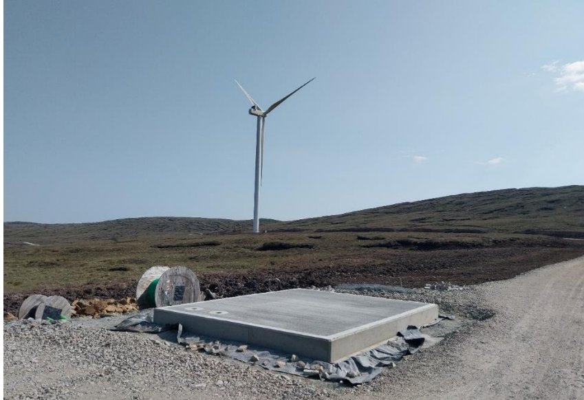
Photo 3. LiDAR Plinth installed by T001
