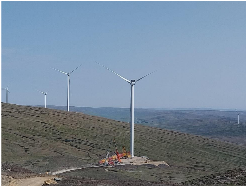
Photo 1. Crane being de-rigged following turbine erection at T026
