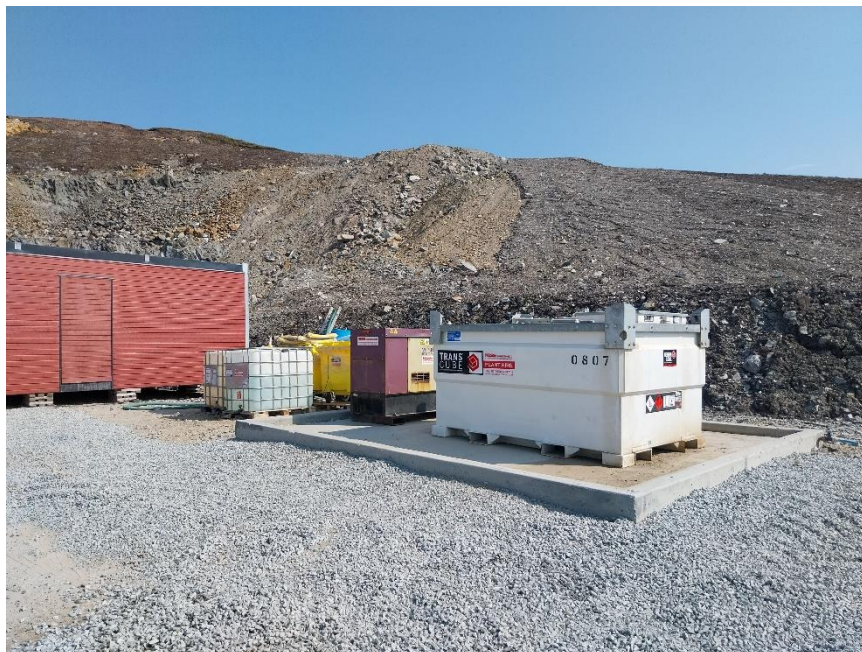
Photo 4. Bunded IBCs and fuel tanks at KBP05 Vestas Satellite Compound
