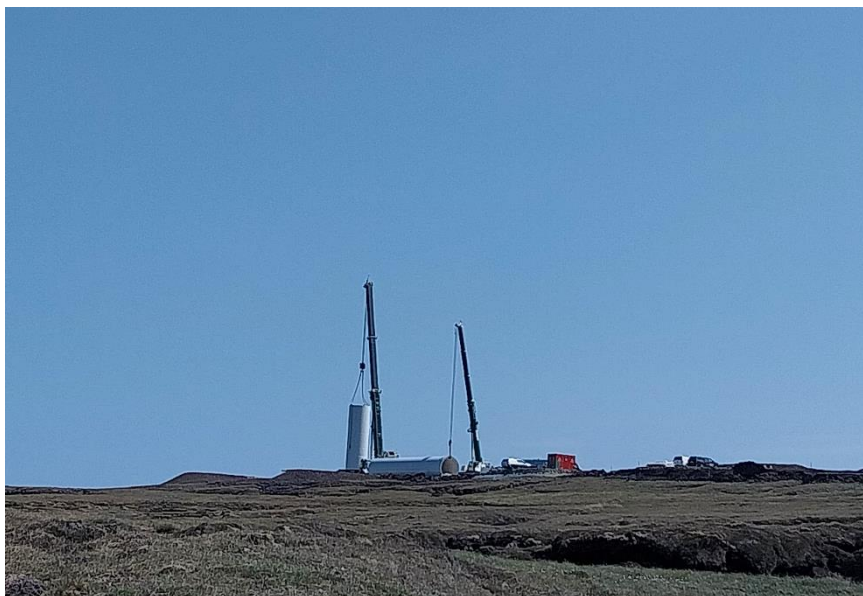
Photo 12. First two sections of tower being lifted at T095
