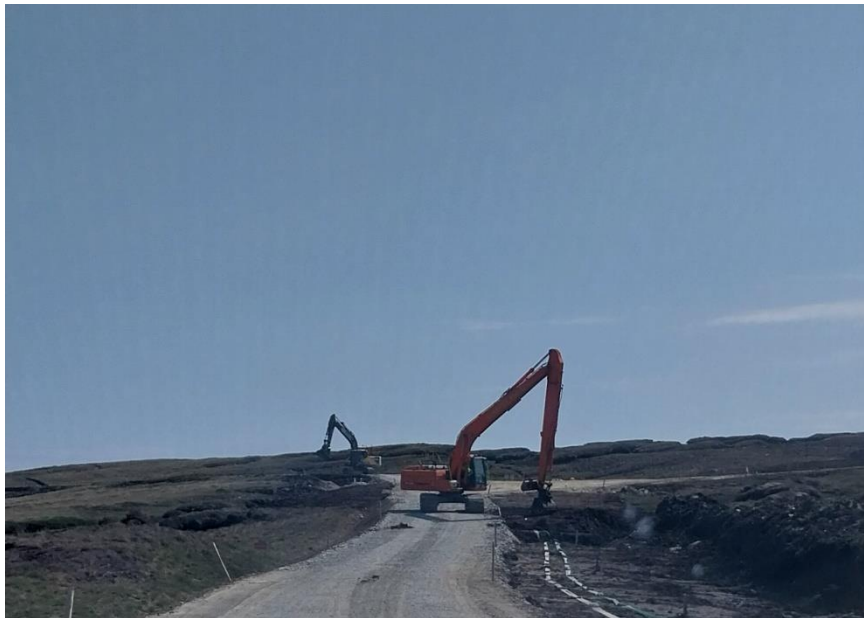
Photo 14. Backfilling of cable trenches by T095
