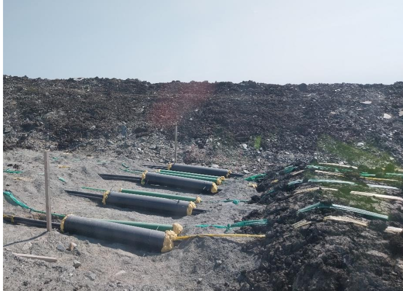
Photo 5. Preparation for concrete plug installation in cable trench by T024
