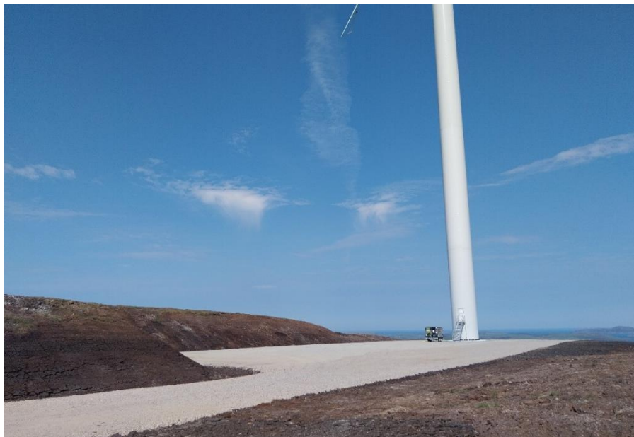
Photo 2. Capped road and hardstanding at T001
