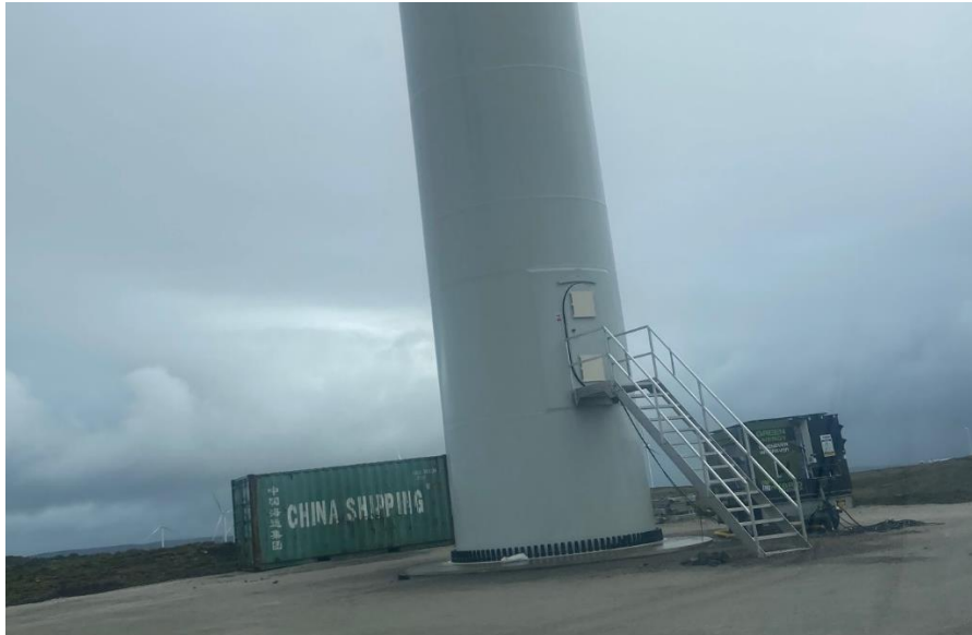
Photo 9. On-going pre-energisation checks at T041
