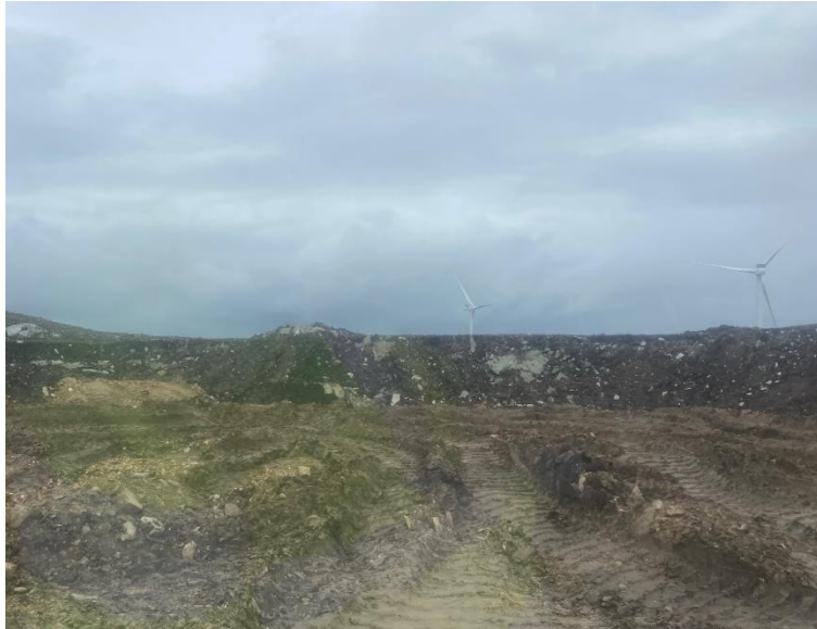
Photo 7. Temporary peat storage at the back of KBP02
