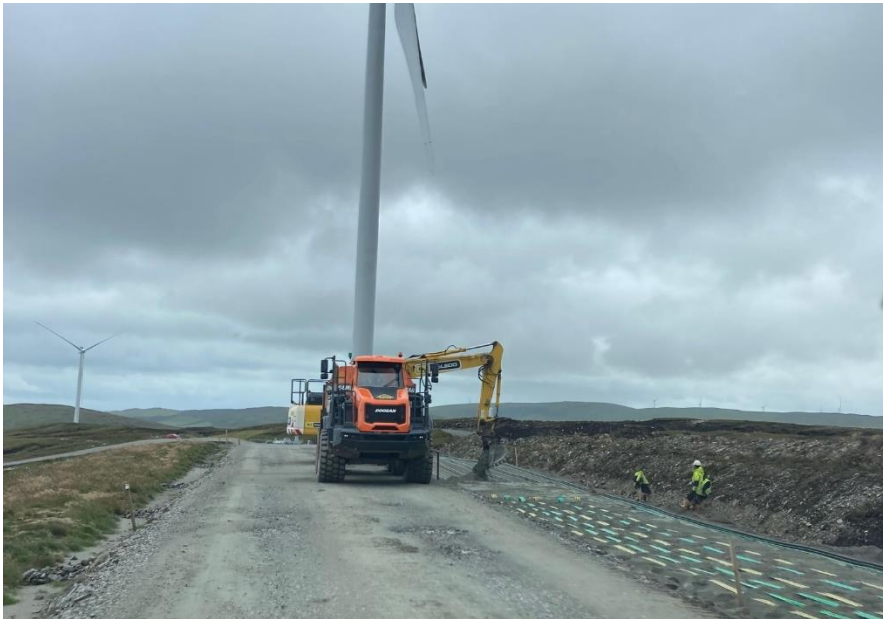
Photo 17. Cable trench backfilling by T071
