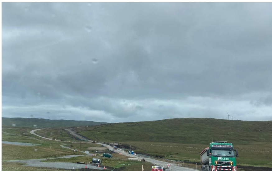
Photo 10. On-going backfilling works along the Sandwater track
