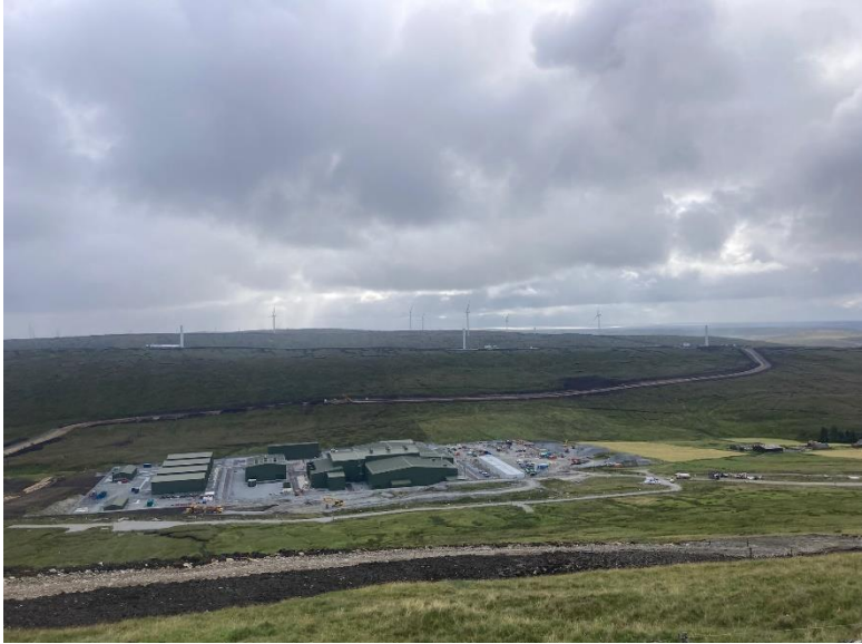
Photo 19. Substation observed from Spur 5 on approach to Upper Kergord
