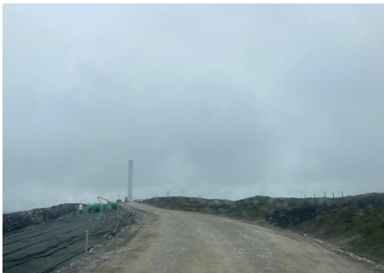
Photo 8. Cable laying and trench backfilling operations south of T036
